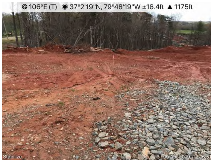
Fig. 3: STA 14354+10 – S-A40: No stabilization on CIS or GAS of S-38/40. No Earth-Guard present.
