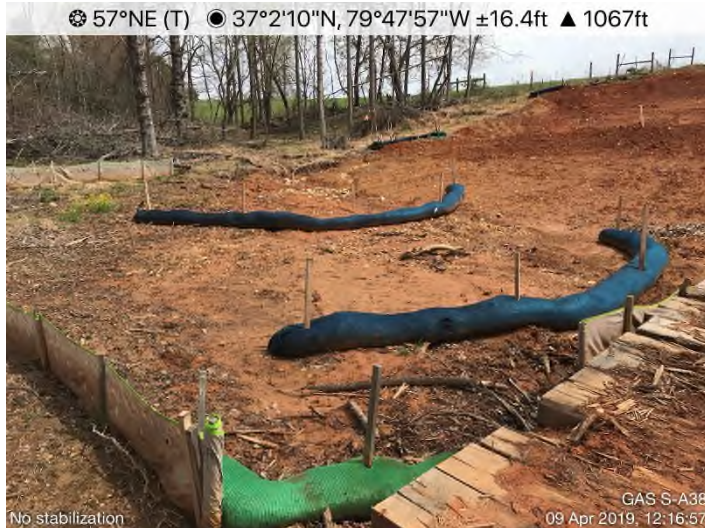
Fig. 3: STA 14354+10 – S-A40: No stabilization on CIS or GAS of S-38/40. No Earth-Guard present.
