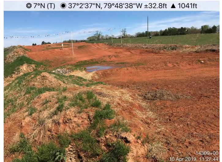
Fig. 4: STA 14309+00 – Area stabilized with Earth-Guard. Controls in place.
