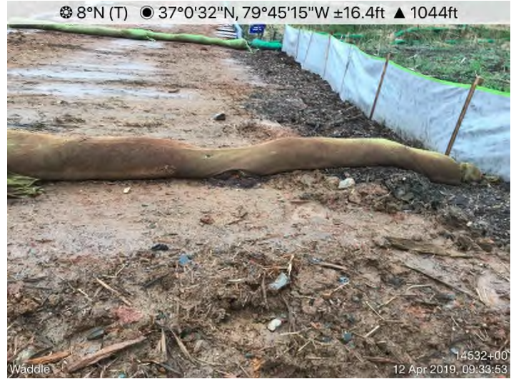
Fig. 4: STA 14533+00 – No inlet protection. Inlet too high.
