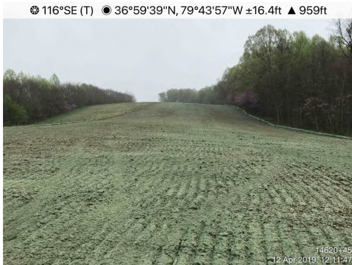
Fig. 7: STA 14644+45 - Area at final stabilization.
