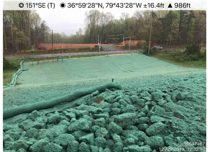
Fig. 8: STA 14647+87 – Area at final stabilization.
