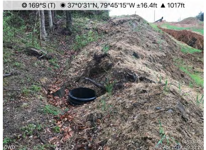
Fig. 4: STA 14533+00 – No inlet protection. Inlet too high.
