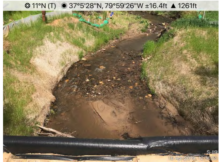
Fig. 12: S-II9 – Controls in place. Banks Stabilized.
