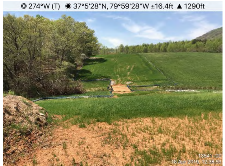
Fig. 12: S-II9 – Controls in place. Banks Stabilized.
