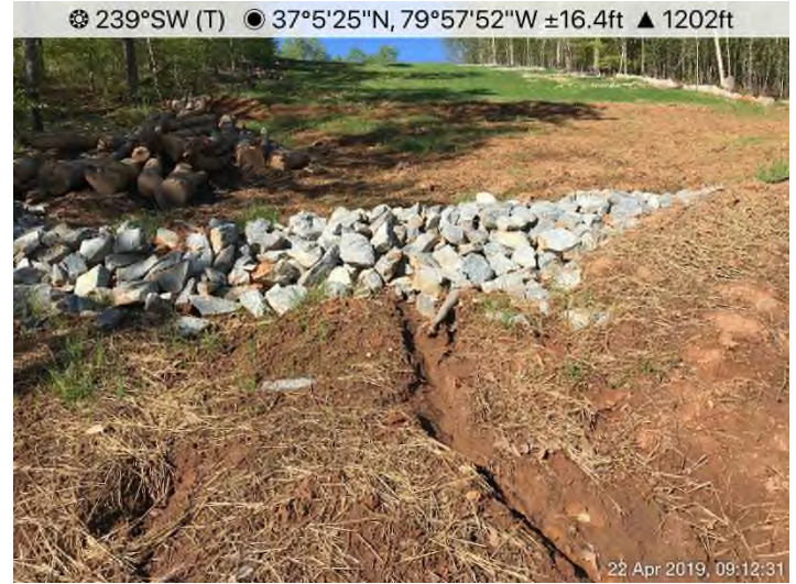
Fig. 4: St. Clair Access Road – Stabilize shoulder of access road.
