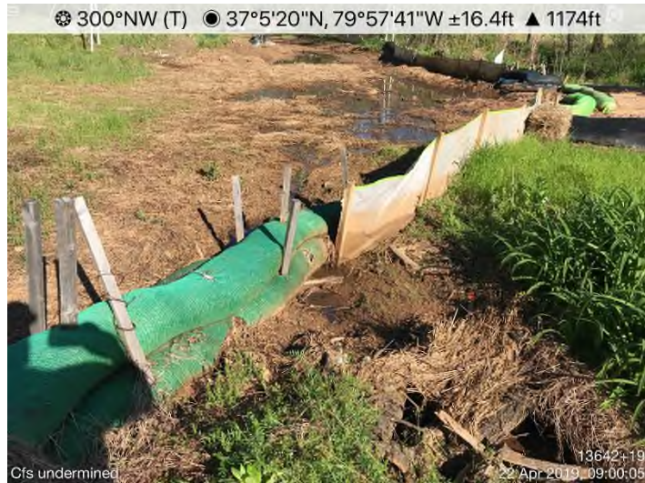
Fig. 3: STA 13630+00 – 13631+50 – Erosion below permanent waterbars.
