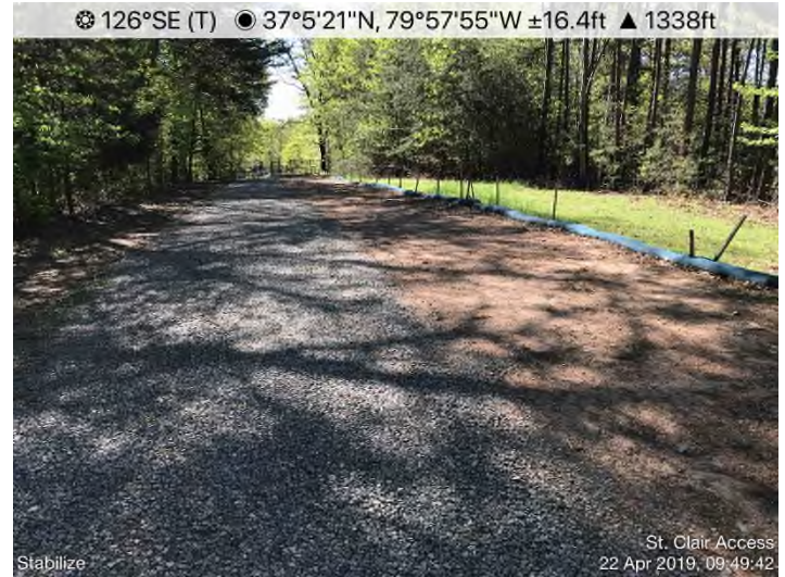
Fig. 4: St. Clair Access Road – Stabilize shoulder of access road.
