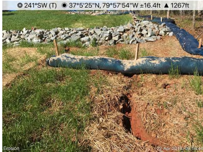
Fig. 3: STA 13630+00 – 13631+50 – Erosion below permanent waterbars.
