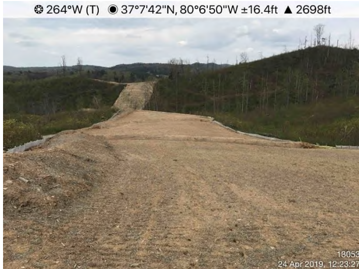
Fig. 7: STA 13053 – Controls in place. Area stabilized with Earth Guard and straw.
