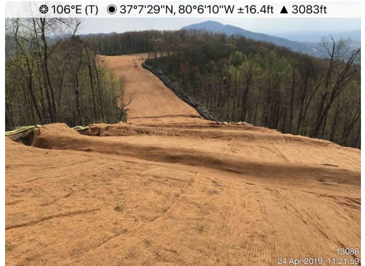
Fig. 4: STA 13086 – Controls in place. Area stabilized with curlex fabric.
