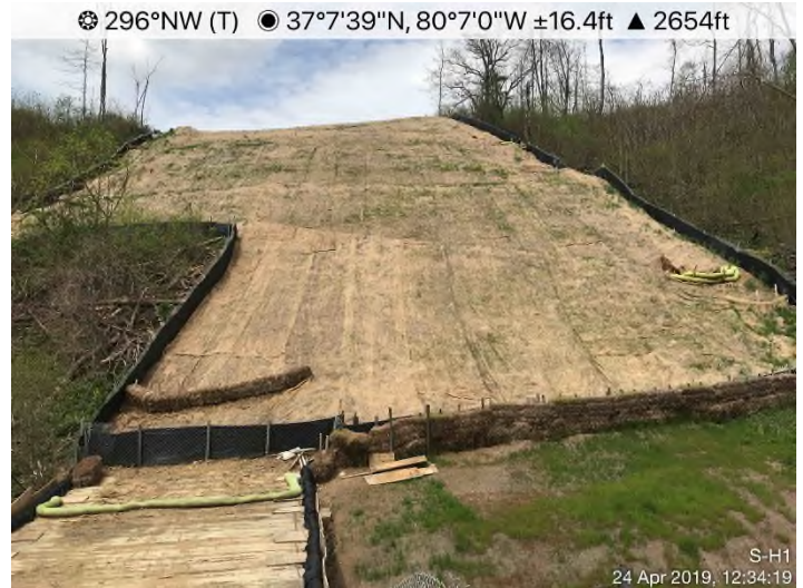
Fig. 8: S-H1 – Controls in place. Area stabilized with curlex fabric.
