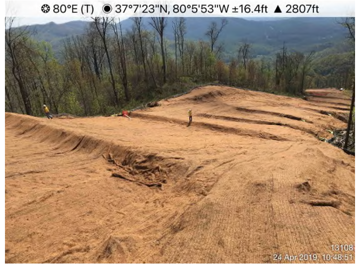
Fig. 4: STA 13086 – Controls in place. Area stabilized with curlex fabric.
