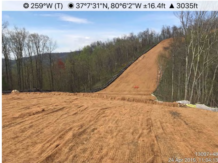
Fig. 3: STA 13097+48 – Controls in place. Area stabilized with curlex fabric.
