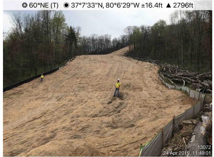
Fig. 8: S-H1 – Controls in place. Area stabilized with curlex fabric.
