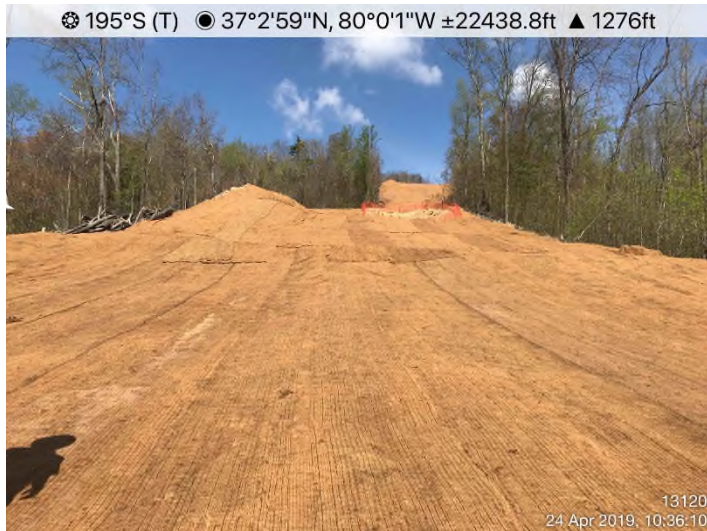
Fig. 3: STA 13097+48 – Controls in place. Area stabilized with curlex fabric.
