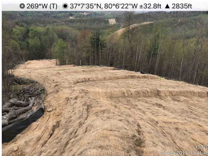
Fig. 7: STA 13053 – Controls in place. Area stabilized with Earth Guard and straw.
