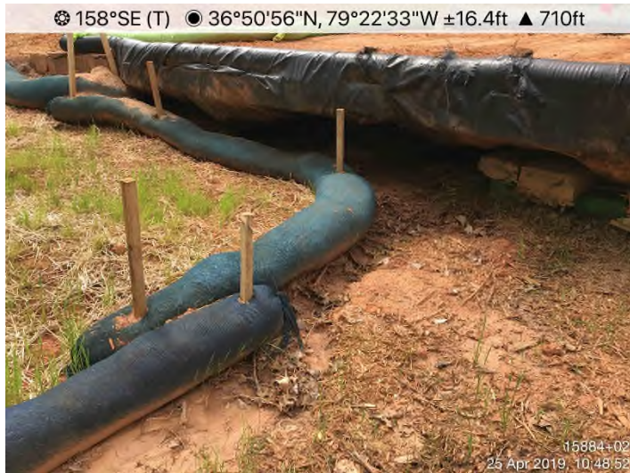
Fig. 3: STA 15922+50 – Sump needs maintenance.
