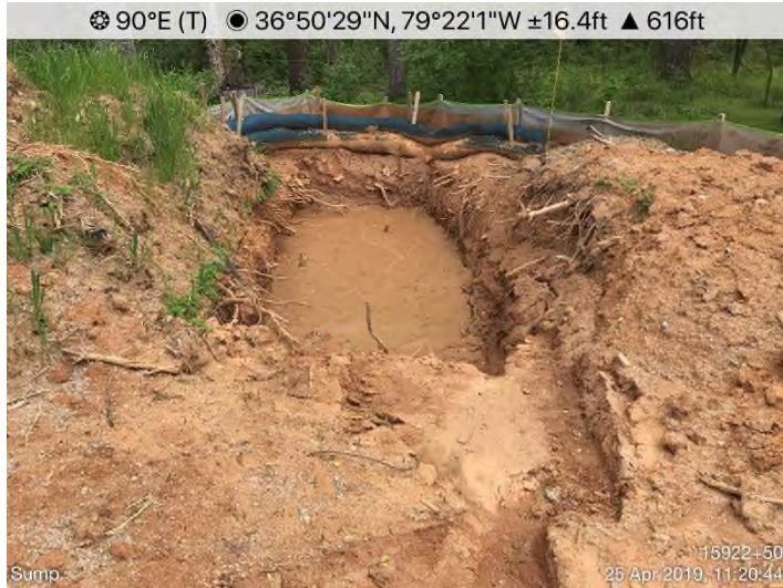
Fig. 3: STA 15922+50 – Sump needs maintenance.
