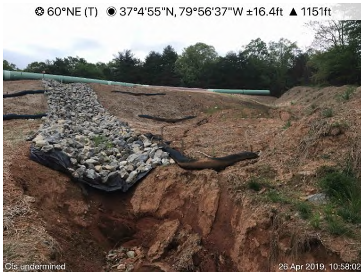
Fig. 7: STA 13712+50 – CFS full, inadequate stabilization.
