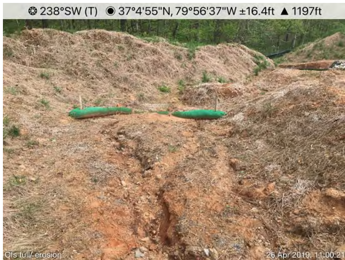
Fig. 7: STA 13712+50 – CFS full, inadequate stabilization.
