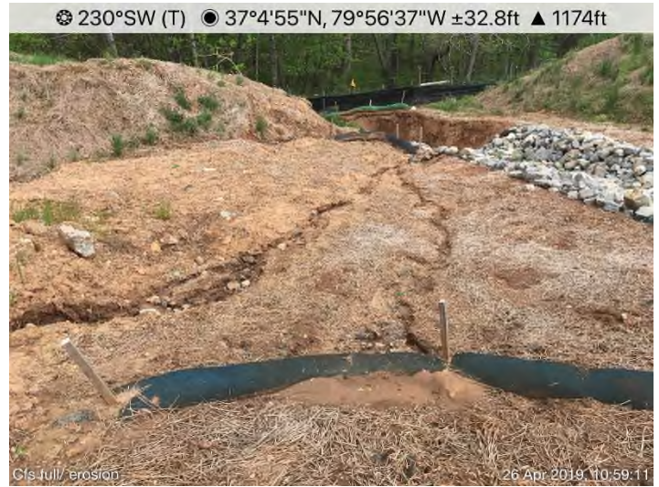
Fig. 8: STA 13717+00 – Area stabilized. Controls in place.
