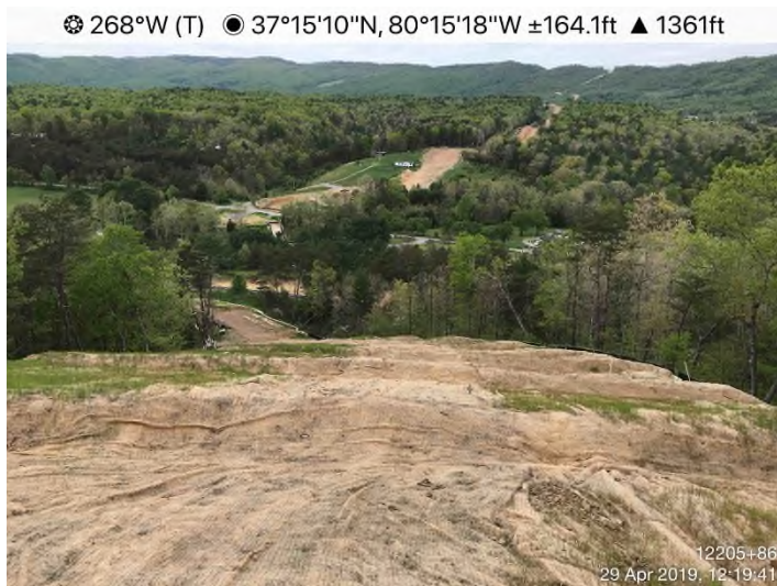
Fig. 7: STA 12187+80 – Controls in place. Area stabilized with straw.
