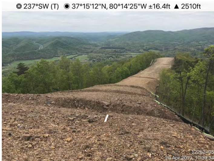
Fig. 3: STA 12218+65 – Controls in place. Area stabilized with Earth Guard.
