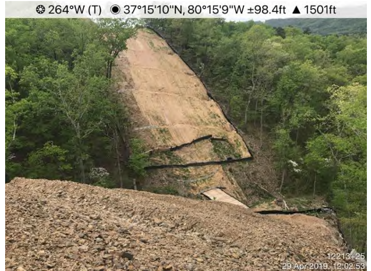
Fig. 4: STA 12213+25 – Controls in place. Area stabilized with curlex fabric and Earth Guard.
