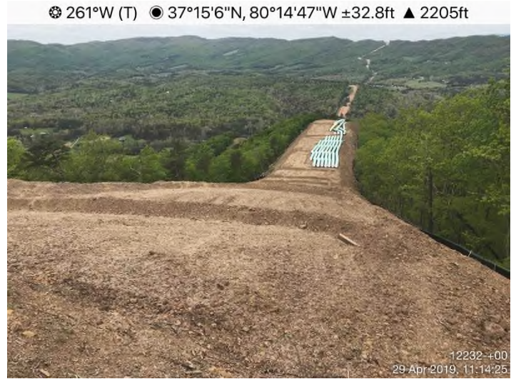
Fig. 4: STA 12213+25 – Controls in place. Area stabilized with curlex fabric and Earth Guard.
