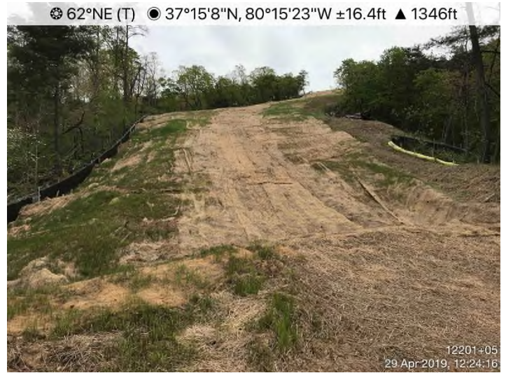
Fig. 8: 12153+00 – Controls in place. Area stabilized with straw.
