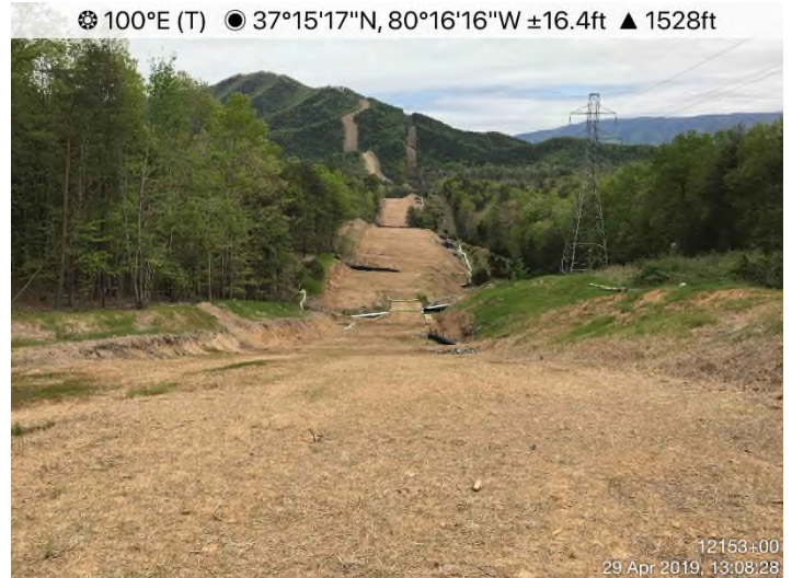
Fig. 8: 12153+00 – Controls in place. Area stabilized with straw.
