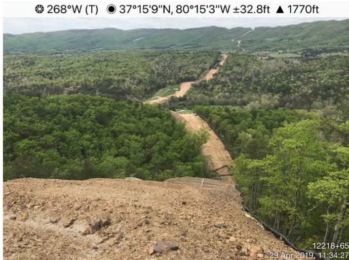
Fig. 3: STA 12218+65 – Controls in place. Area stabilized with Earth Guard.
