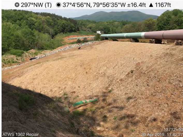
Fig. 7: STA 13712+50 – Area stabilized with straw and curlex.
