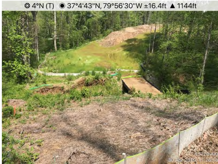
Fig. 3: STA 13720+00 – Controls in place. Area stabilized.
