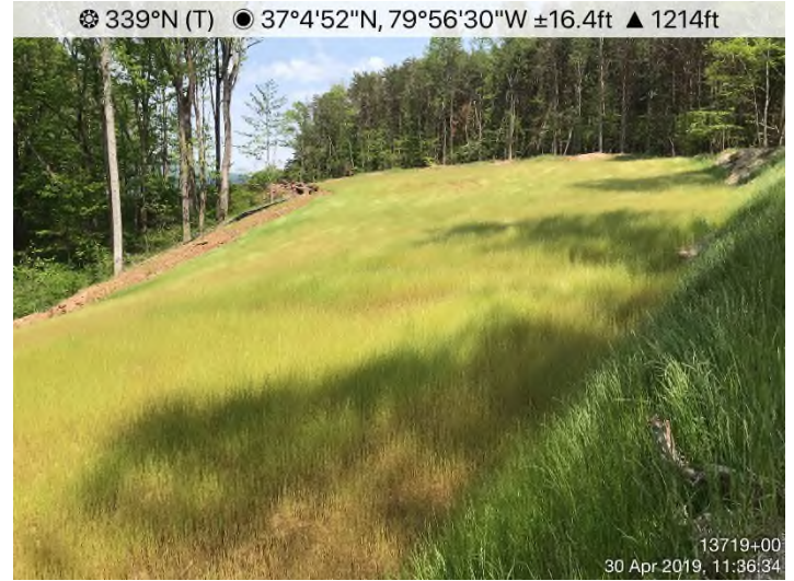
Fig. 8: STA 13712+50 – Area stabilized with straw and curlex.
