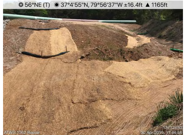
Fig. 8: STA 13712+50 – Area stabilized with straw and curlex.
