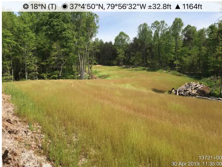
Fig. 7: STA 13712+50 – Area stabilized with straw and curlex.
