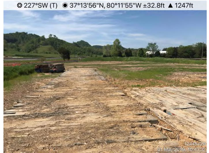
Fig. 4: STA 12445+29 – Controls in place. Area stabilized.
