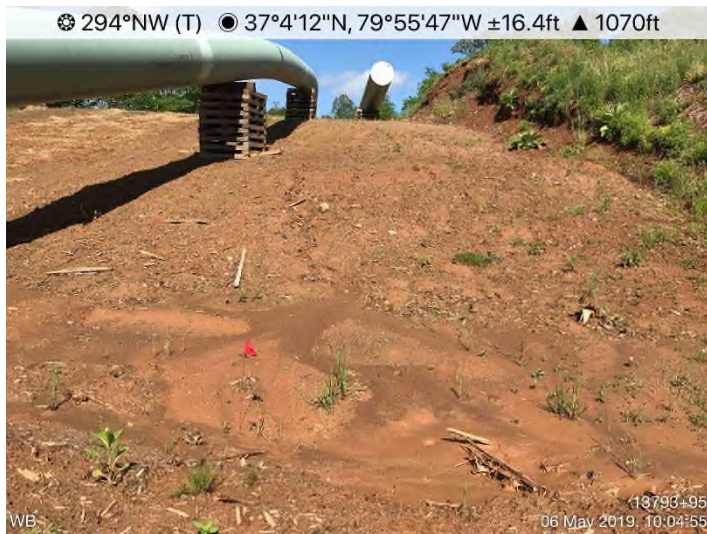
Fig. 3: STA 13793+95 – Stabilize area upslope of waterbar.
