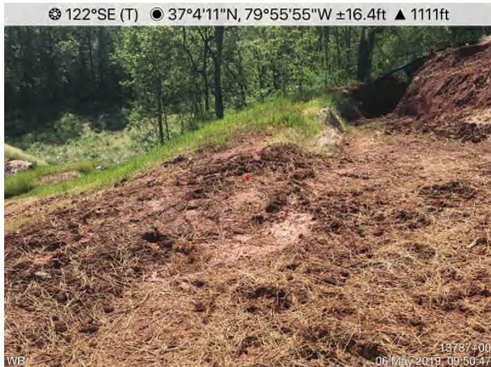
Fig. 3: STA 13793+95 – Stabilize area upslope of waterbar.
