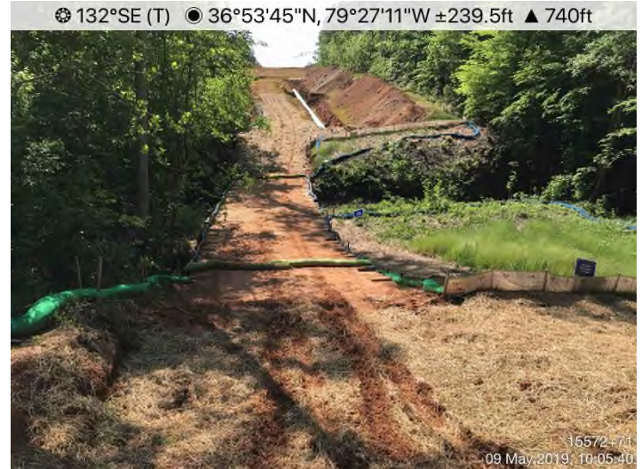
Fig. 4: STA 15556+23 – P1 not properly entrenched.
