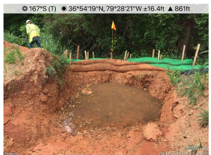
Fig. 8: STA 15505+00 – Sump maintenance needed.
