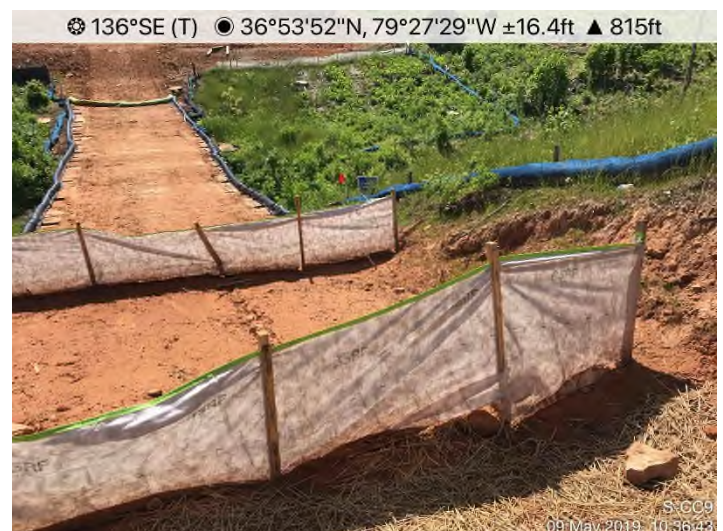
Fig. 4: STA 15556+23 – P1 not properly entrenched.
