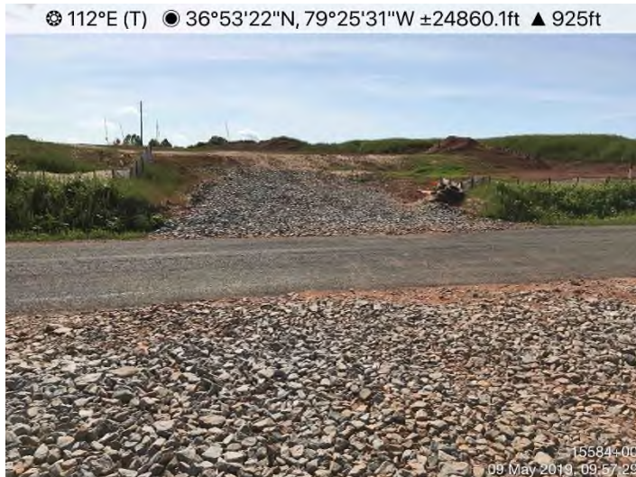
Fig. 3: STA 15562+25 – CFS in need of maintenance.
