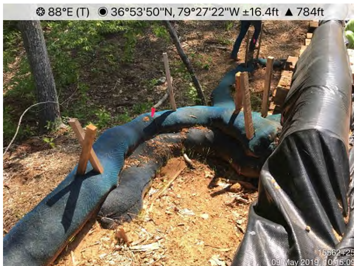
Fig. 3: STA 15562+25 – CFS in need of maintenance.
