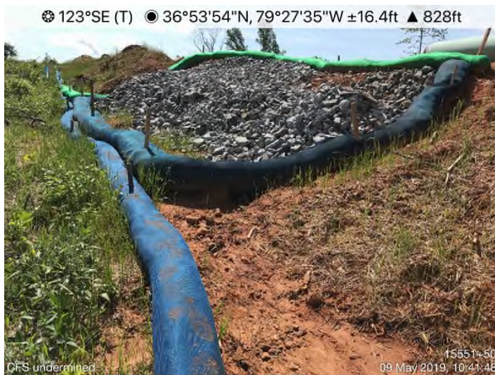
Fig. 7: STA 15514+00 - 15515+00 – CFS maintenance needed.
