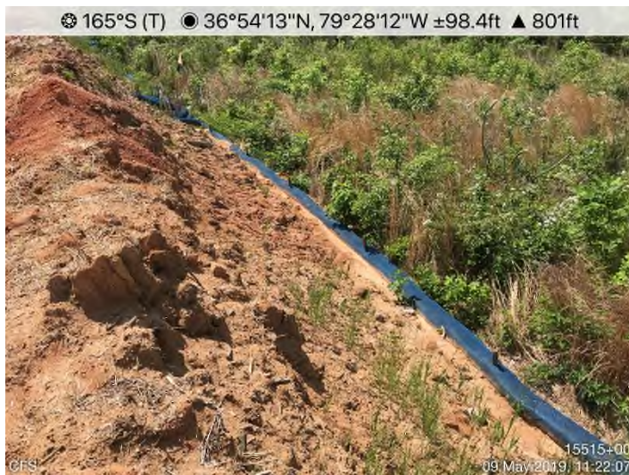
Fig. 7: STA 15514+00 - 15515+00 – CFS maintenance needed.
