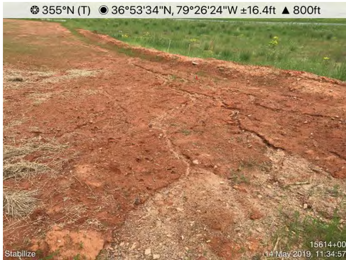
Fig. 3: STA 15614+00 – Inadequate stabilization.
