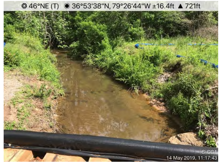
Fig. 8: STA 15615+12 – Controls in place. Area adequately stabilized with straw and Earth Guard.
