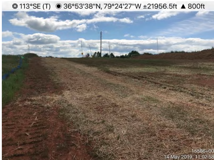
Fig. 3: STA 15614+00 – Inadequate stabilization.
