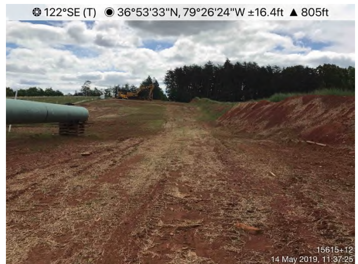
Fig. 8: STA 15615+12 – Controls in place. Area adequately stabilized with straw and Earth Guard.
