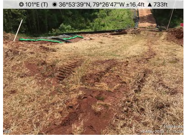
Fig. 4: STA 15623+00 – CFS undermined.
