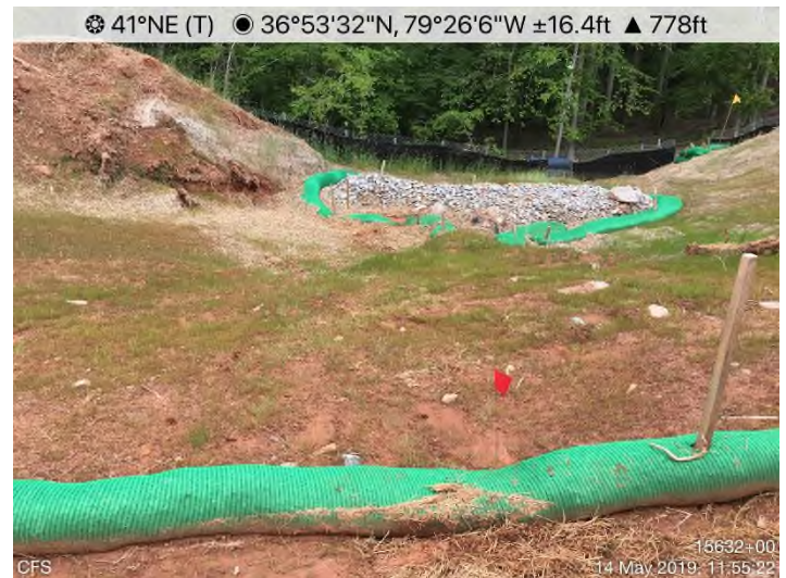
Fig. 4: STA 15623+00 – CFS undermined.
