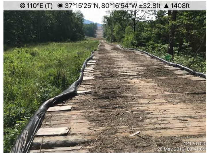
Fig. 4: STA 12171+00 – Controls in place. Area stabilized with erosion fabric, Earth Guard and straw.
