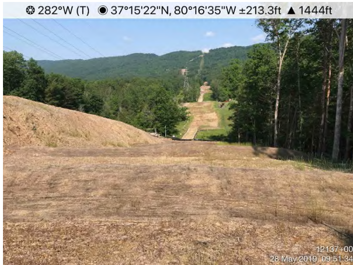
Fig. 3: STA 12137+00 – Controls in place. Area stabilized with erosion fabric, Earth Guard and straw.
