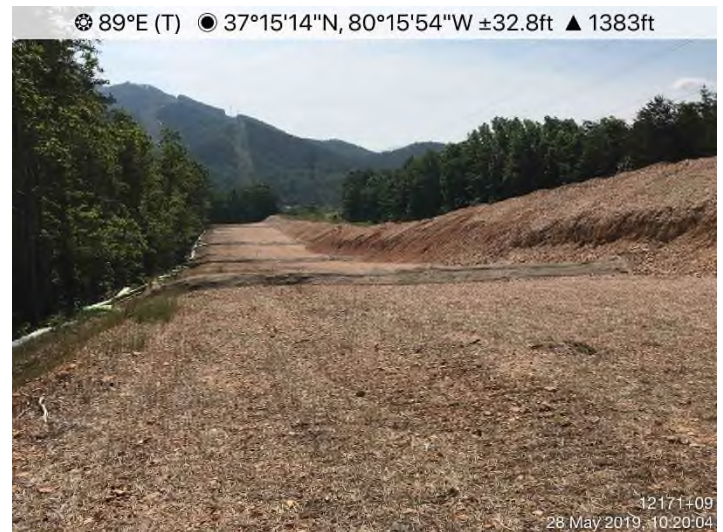
Fig. 4: STA 12171+00 – Controls in place. Area stabilized with erosion fabric, Earth Guard and straw.
