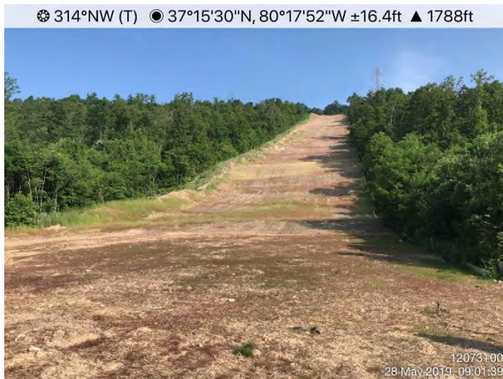
Fig. 3: STA 12137+00 – Controls in place. Area stabilized with erosion fabric, Earth Guard and straw.
