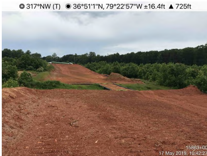
Fig. 3: STA 15863+00 – Controls in place. Area stabilized with Earth Guard.
