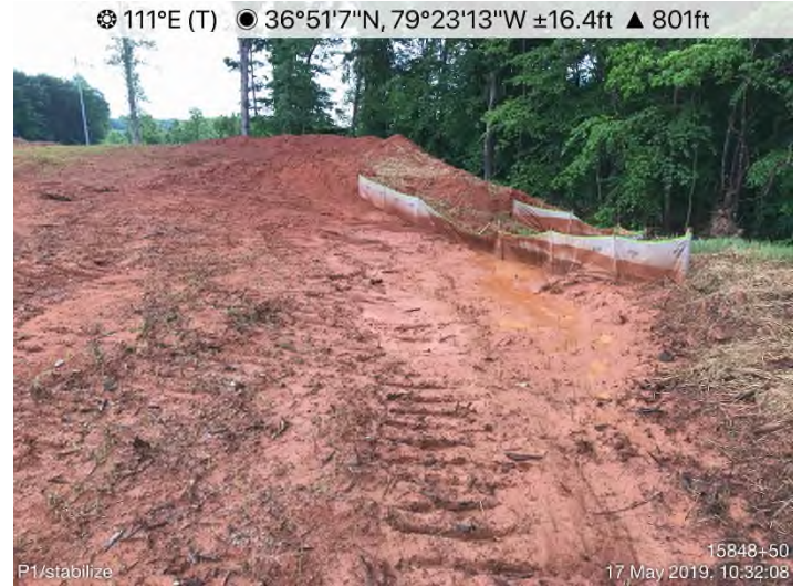
Fig. 4: STA 15868+70 – Sediment off ROW. Upgrade ECDs/repair as needed.
