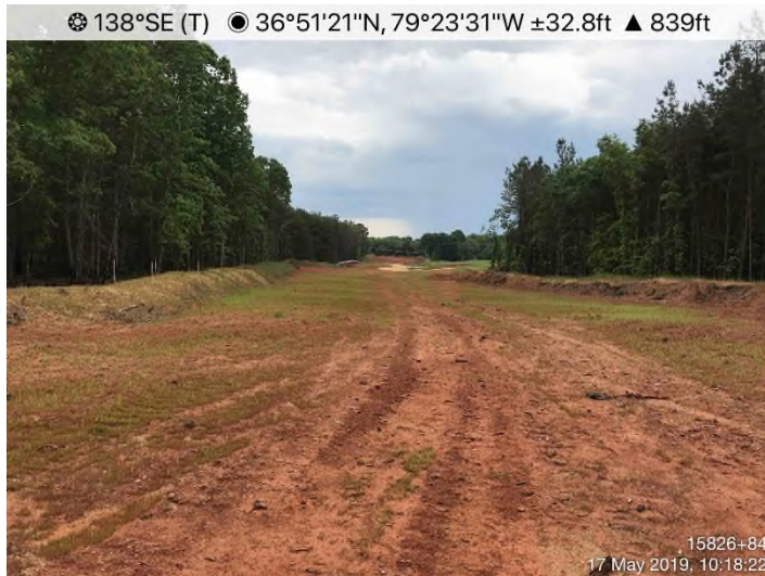
Fig. 3: STA 15863+00 – Controls in place. Area stabilized with Earth Guard.
