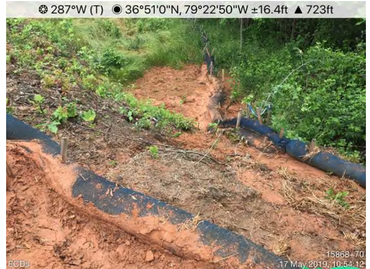
Fig. 4: STA 15868+70 – Sediment off ROW. Upgrade ECDs/repair as needed.
