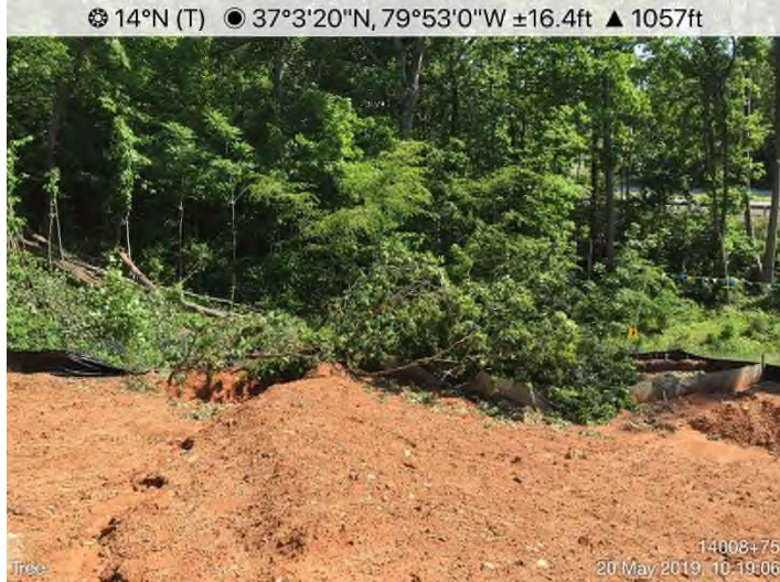
Fig. 3: STA 14008+75 – Remove fallen tree. Repair ECDs.
