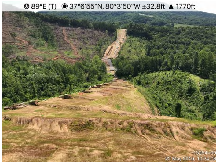
Fig. 7: STA 13303+00 – Controls in place. Area stabilized with erosion fabric/Earth Guard.
