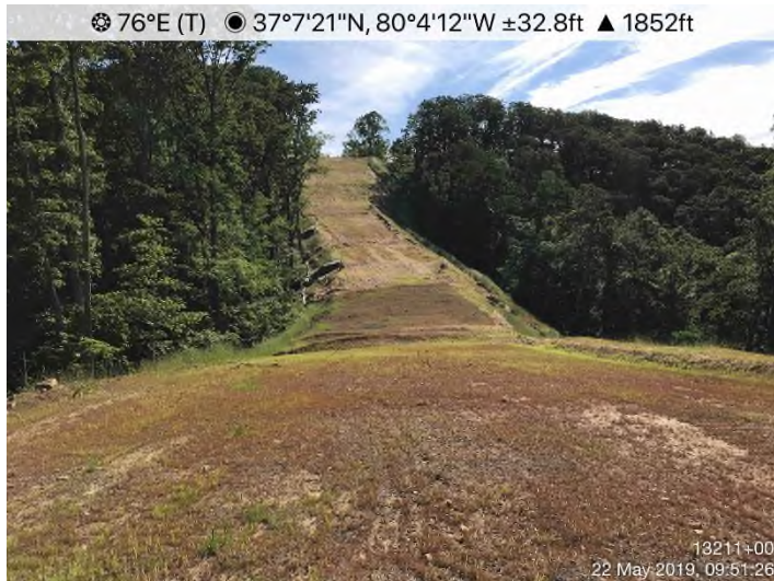
Fig. 3: STA 13236+00 – Controls in place. Area stabilized with erosion fabric/Earth Guard.
