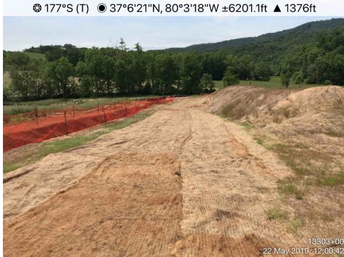
Fig. 7: STA 13303+00 – Controls in place. Area stabilized with erosion fabric/Earth Guard.
