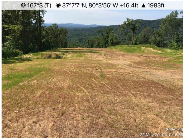
Fig. 3: STA 13236+00 – Controls in place. Area stabilized with erosion fabric/Earth Guard.
