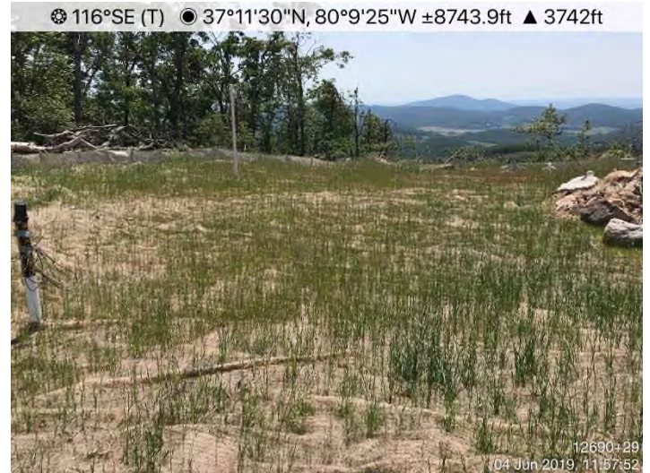
Fig. 4: STA 12690+29 – Controls in place. Area stabilized with fabric.
