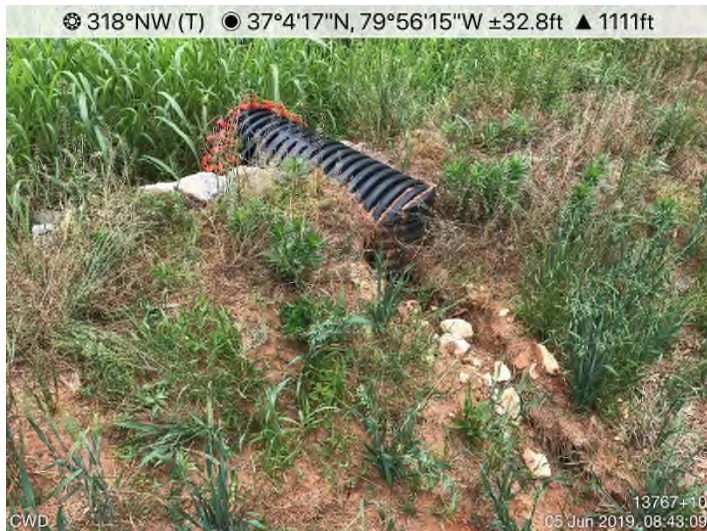
Fig. 3: STA 13793+96 – Sump maintenance needed.
