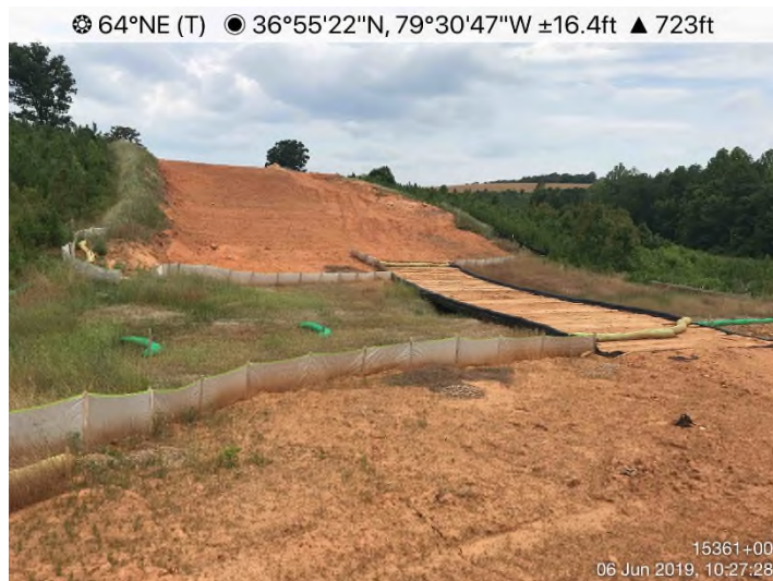
Fig. 3: STA 15442+00 – Controls in place. Area stabilized with straw and Earth-Guard.
