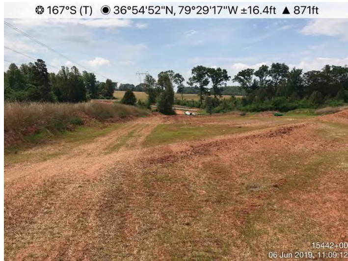
Fig. 3: STA 15442+00 – Controls in place. Area stabilized with straw and Earth-Guard.
