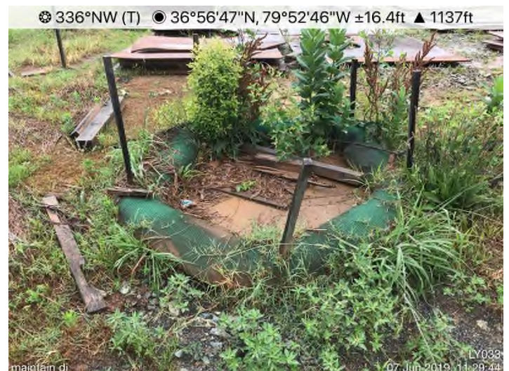
Fig. 4: Laydown Yard 033 – Drop inlet maintenance needed.
