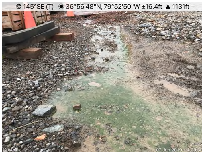
Fig. 3: Laydown Yard 032 – Runoff contaminated with fertilizer.
