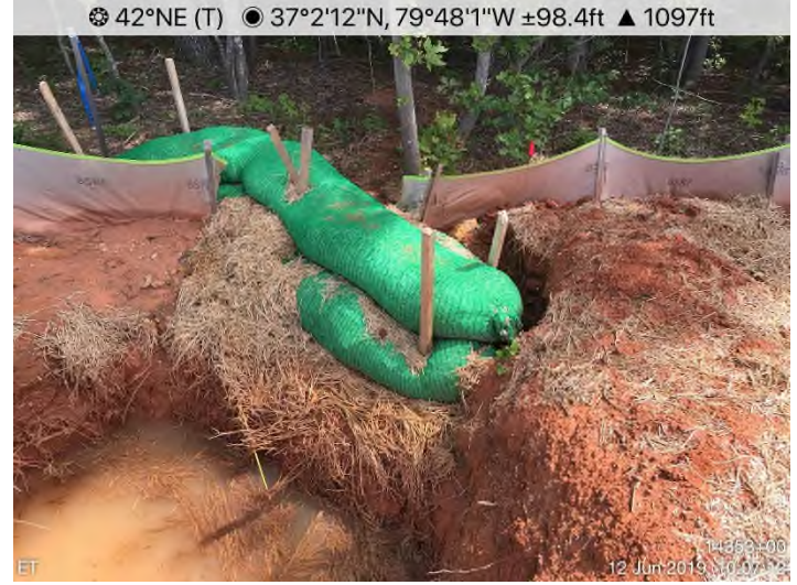
Fig. 4: STA 14351+00 to 14352+00 – P1 undermined.
