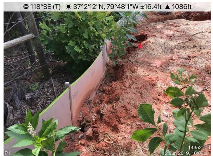
Fig. 4: STA 14351+00 to 14352+00 – P1 undermined.
