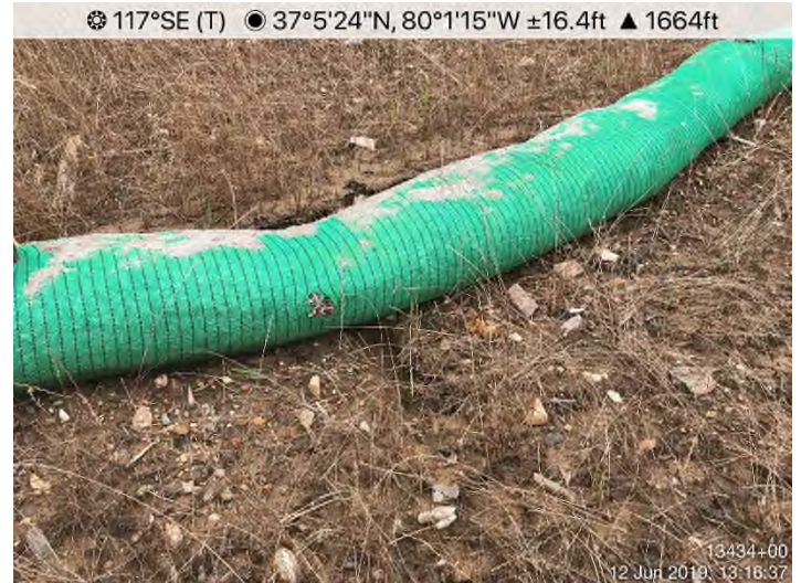
Fig. 8: STA 13434+00 – CFS undermined.
