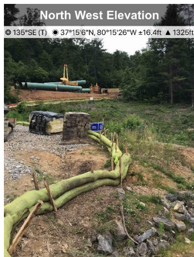
Fig. 3. ECD controls are in place at designated stream S-001
