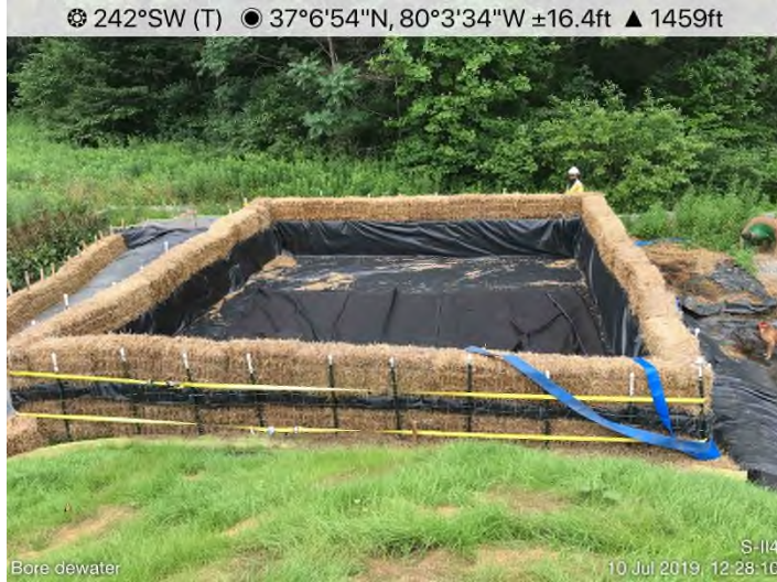
Fig. 3: ATWS 1055 – Dewatering structure for GAS of conventional bore pit. Sediment bags are clean, filter structure intact and dewatering to stabilized area.
