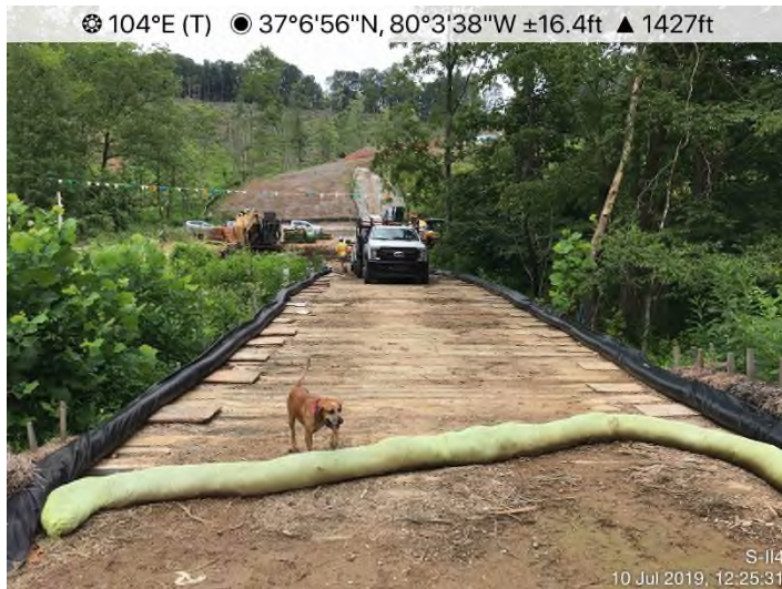
Fig. 3: ATWS 1055 – Dewatering structure for GAS of conventional bore pit. Sediment bags are clean, filter structure intact and dewatering to stabilized area.
