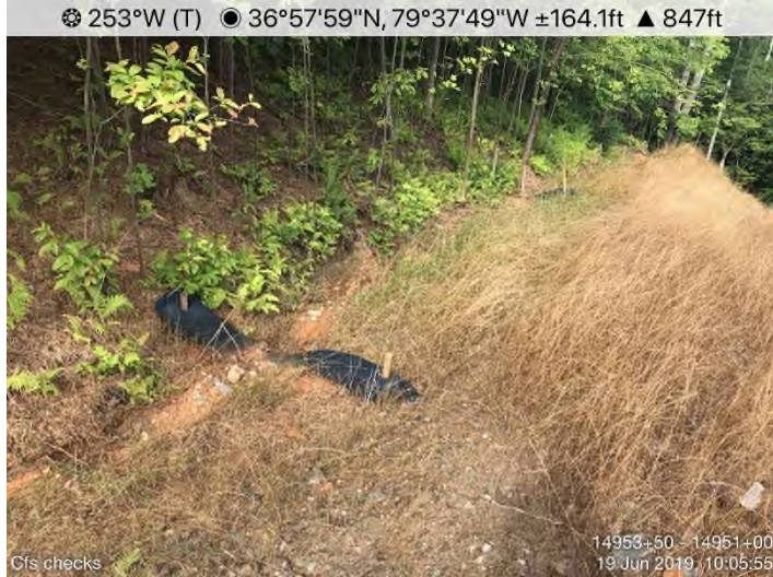
Fig. 7: STA 14951+00 to 14953+50 – CFS maintenance needed.
