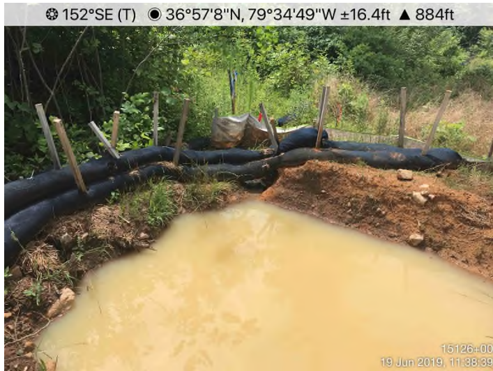
Fig. 11: STA 15126+00 – CFS/P1 maintenance needed.
