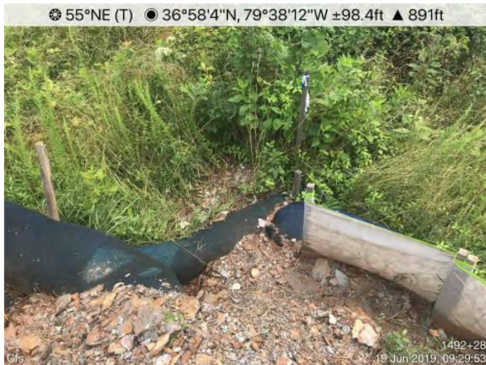
Fig. 3: STA 14943+00 – CFS maintenance needed. Repair and stabilize diversion berm.
