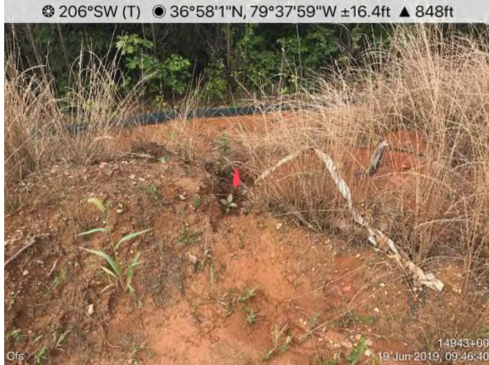
Fig. 3: STA 14943+00 – CFS maintenance needed. Repair and stabilize diversion berm.
