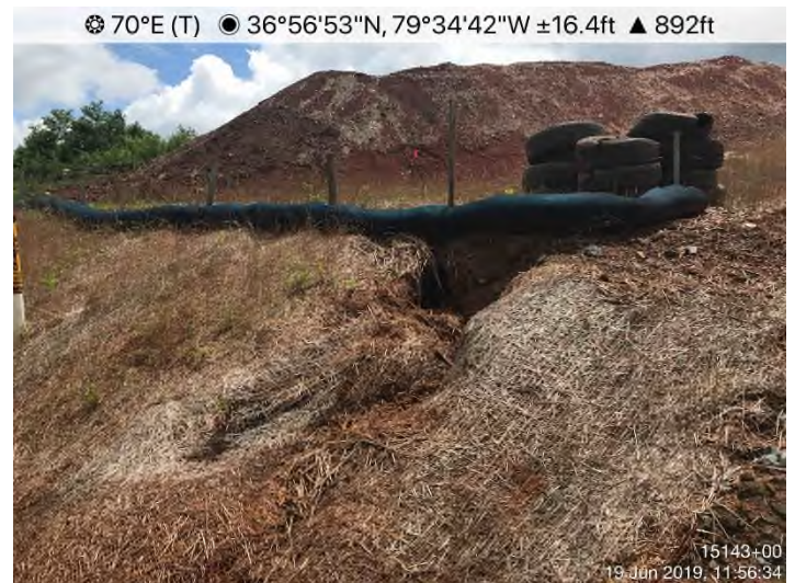
Fig. 12: STA 15143+00 – CFS maintenance needed.
