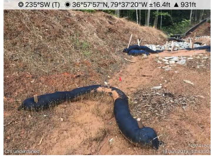
Fig. 12: STA 15143+00 – CFS maintenance needed.
