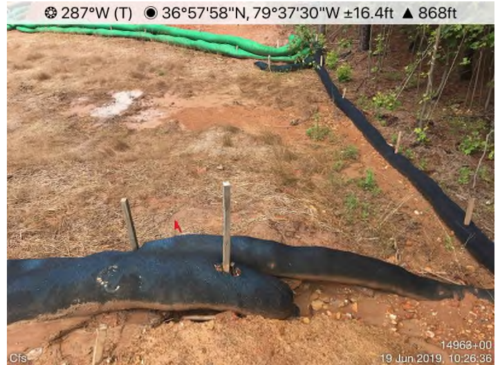
Fig. 8: STA 14967+00 – CFS maintenance needed.
