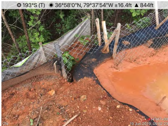
Fig. 7: STA 14951+00 to 14953+50 – CFS maintenance needed.
