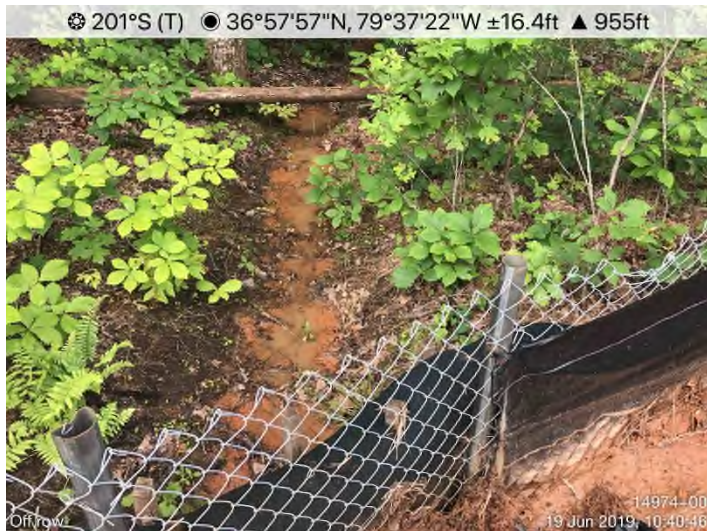
Fig. 11: STA 15126+00 – CFS/P1 maintenance needed.
