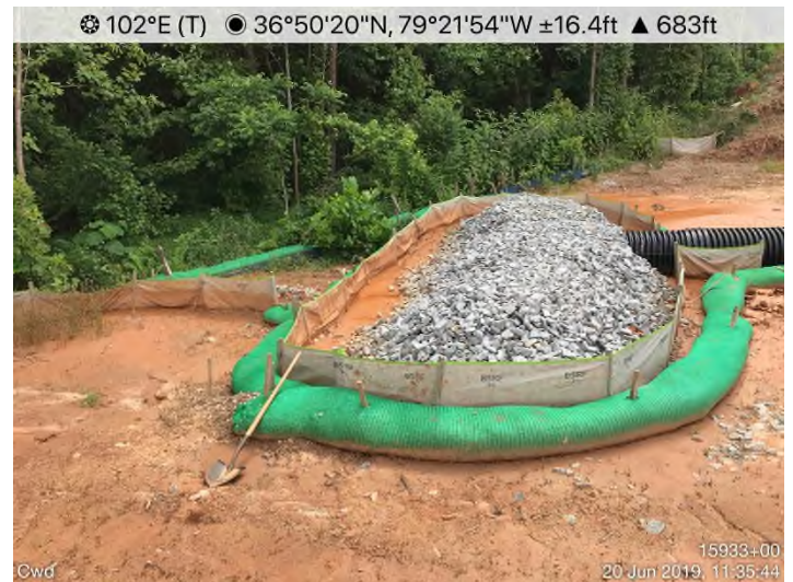
Fig. 8: STA 15933+00 – Sediment accumulation inside CWD outlet. Inadequate protection from onsite discharge.
