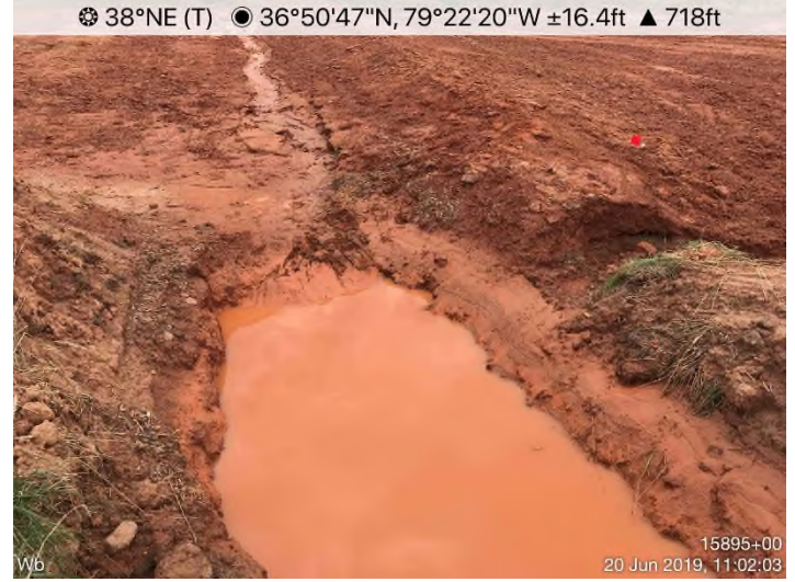
Fig. 8: STA 15933+00 – Sediment accumulation inside CWD outlet. Inadequate protection from onsite discharge.
