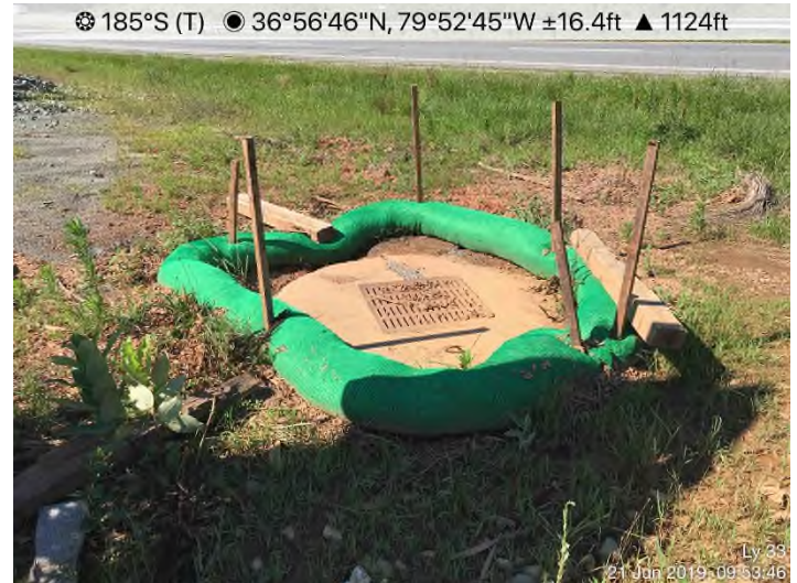
Fig. 4: STA 15737+00 – Controls in place. Area stabilized with Earth-Guard and temp. seed.
