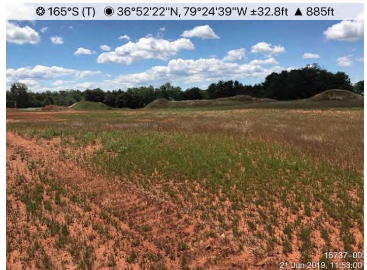
Fig. 4: STA 15737+00 – Controls in place. Area stabilized with Earth-Guard and temp. seed.
