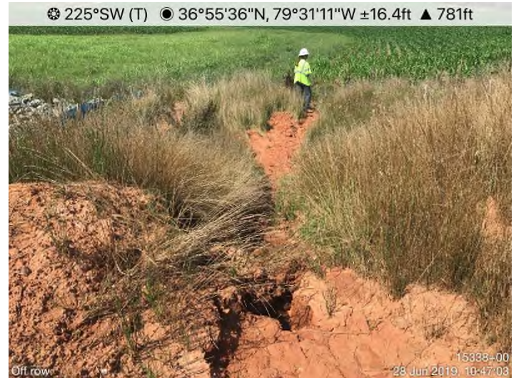
Fig. 8: STA 15345+00 – Sump maintenance needed.
