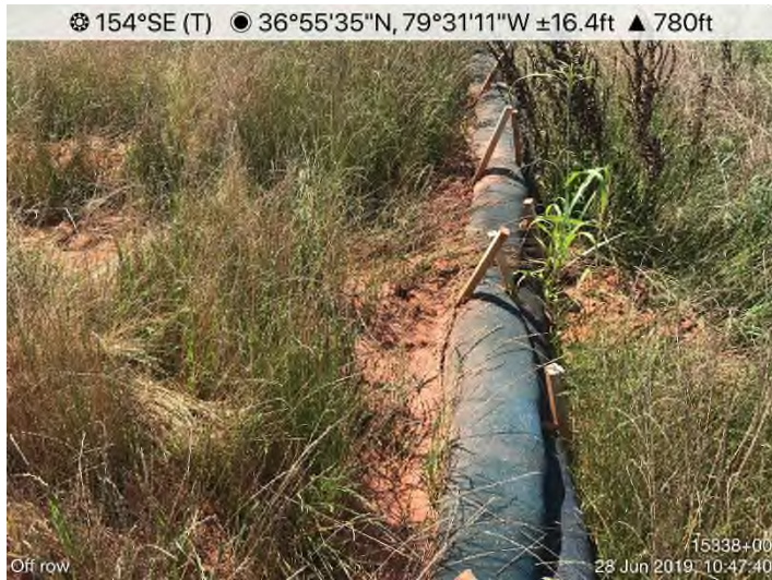
Fig. 7: STA 15338+00 – CFS maintenance needed.
