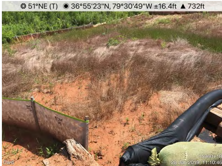
Fig. 9: STA 15360+18 – Onsite sediment discharging into CWD swale.
