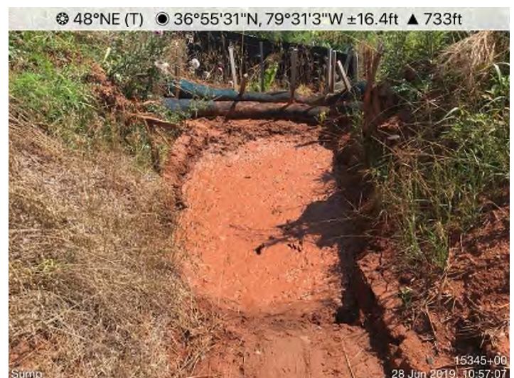
Fig. 8: STA 15345+00 – Sump maintenance needed.
