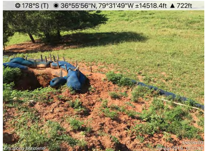
Fig. 4: STA 15310+00 to 15370+00 – Re-stabilization needed.
