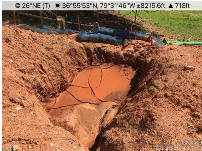
Fig. 3: STA 15333+00 – Sump maintenance needed.
