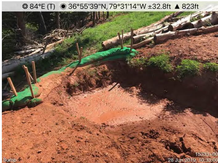
Fig. 3: STA 15333+00 – Sump maintenance needed.
