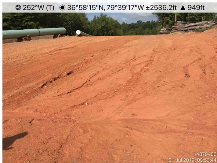
Fig. 3: STA 14861+00 to 14928+00 – Inadequate stabilization.
