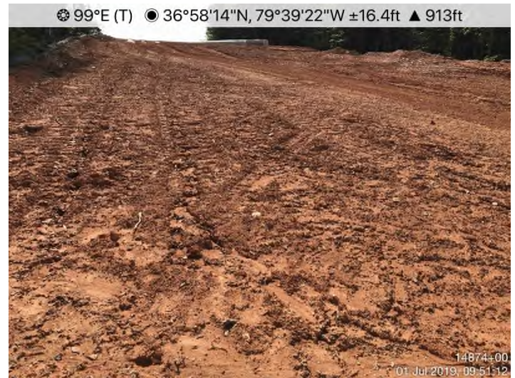
Fig. 4: STA 14861+00 to 14928+00 – Inadequate stabilization.
