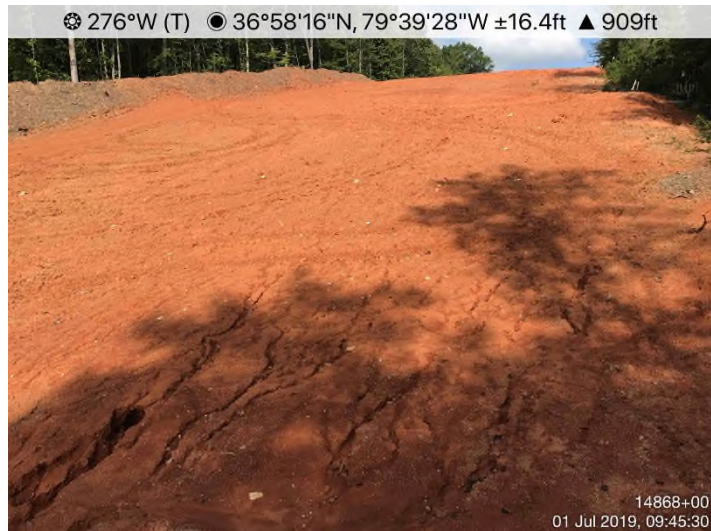
Fig. 3: STA 14861+00 to 14928+00 – Inadequate stabilization.
