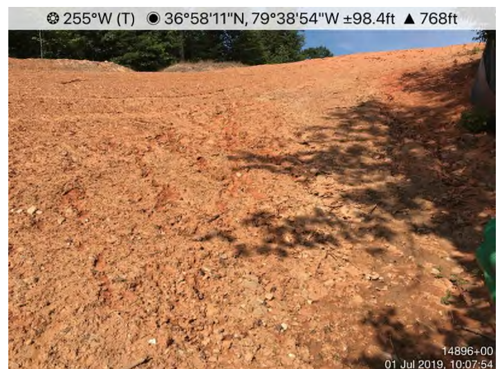
Fig. 4: STA 14861+00 to 14928+00 – Inadequate stabilization.
