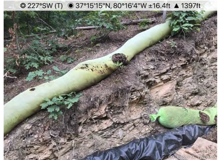
Fig. 4: STA 12163+05 – CFS needs maintenance at stream S-C25.
