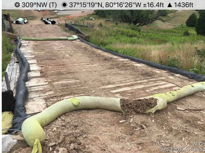
Fig. 3: STA 12143+59 – CFS "Waddles" need maintenance at wetland W-C5.
