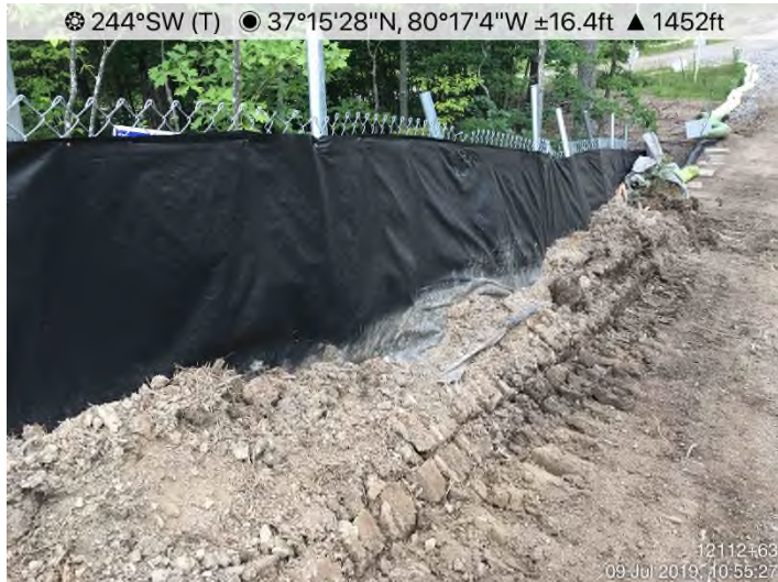
Fig. 3: STA 12143+59 – CFS "Waddles" need maintenance at wetland W-C5.
