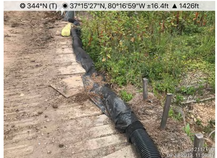
Fig. 4: STA 12163+05 – CFS needs maintenance at stream S-C25.
