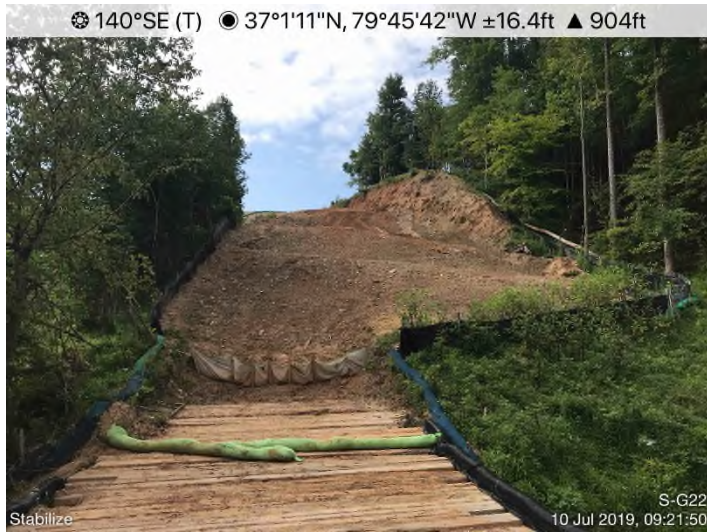
Fig. 3: STA 14485+00 to 14490+00 – Inadequate stabilization.
