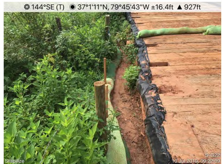
Fig. 4: STA 14485+00 to 14490+00 – Inadequate stabilization.
