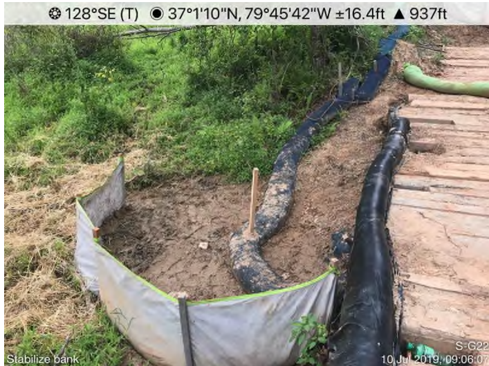
Fig. 3: STA 14485+00 to 14490+00 – Inadequate stabilization.
