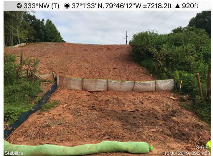
Fig. 4: STA 14485+00 to 14490+00 – Inadequate stabilization.
