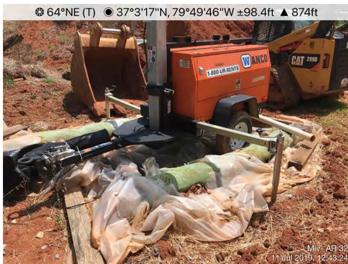
Fig. 7: MVP-MLV-AR-23 – Repair secondary containment structure.
