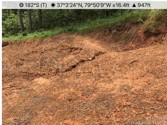
Fig. 3: STA 14217+00 – End treatment undermined.
