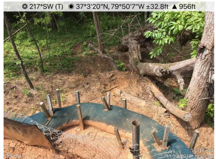
Fig. 4: STA 14217+00 – Sump maintenance needed.
