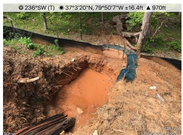
Fig. 4: STA 14217+00 – Sump maintenance needed.
