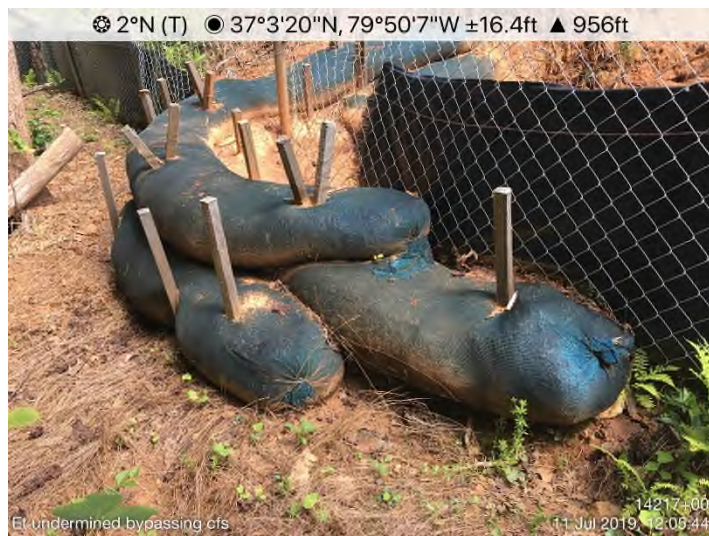
Fig. 3: STA 14217+00 – End treatment undermined.
