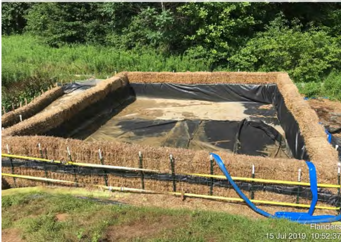
Fig. 3: ATWS 1055 – Dewatering structure for GAS of conventional bore pit. Sediment bags are clean, filter structure intact and dewatering to stabilized area.
