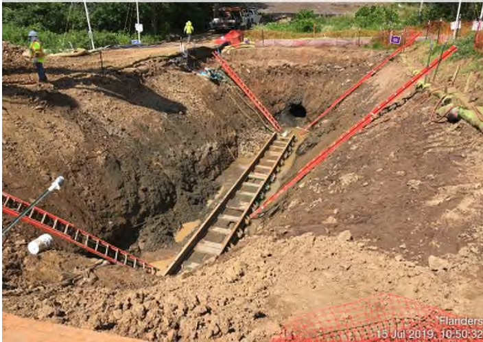
Fig. 3: ATWS 1055 – Dewatering structure for GAS of conventional bore pit. Sediment bags are clean, filter structure intact and dewatering to stabilized area.
