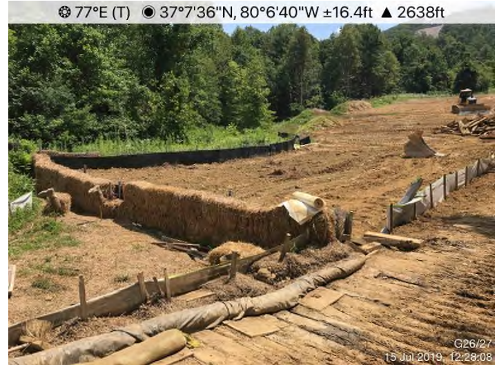
Fig. 8: ATWS 344 – CFS repairs needed. Sump inadequate sizing.
