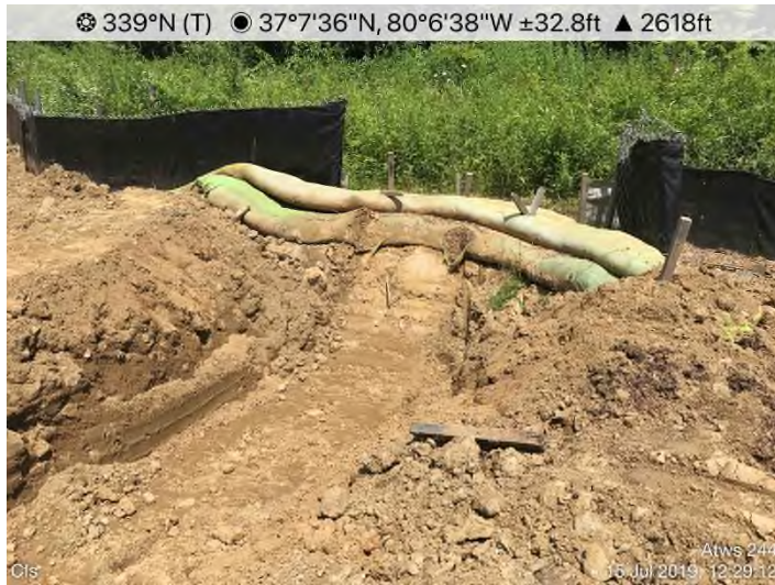
Fig. 7: ATWS 344 – CFS repairs needed.
