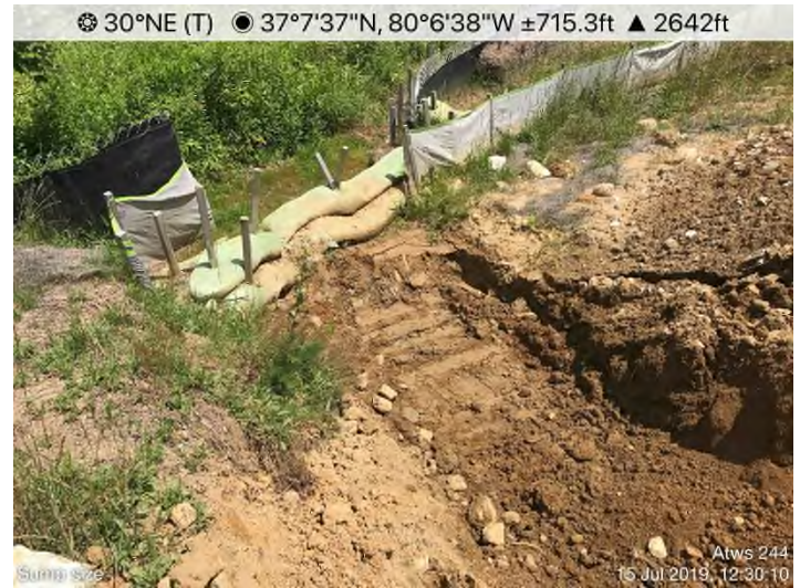
Fig. 8: ATWS 344 – CFS repairs needed. Sump inadequate sizing.
