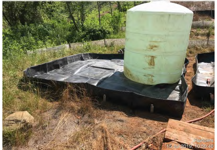
Fig. 4: STA 13262+25 – Secondary containment structures intact and functioning as designed.
