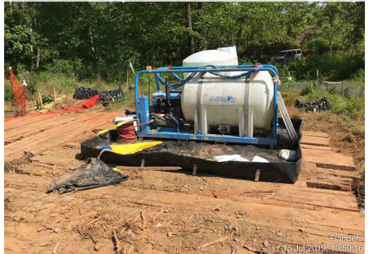
Fig. 4: STA 13262+25 – Secondary containment structures intact and functioning as designed.
