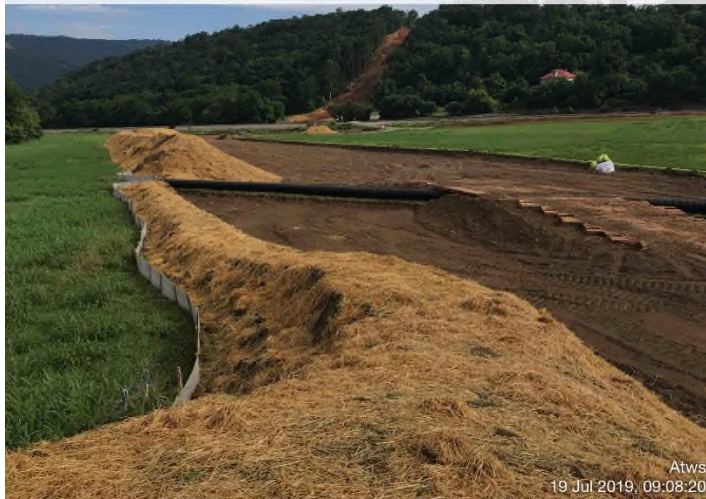
Fig. 3: ATWS 726 – Controls in place and functioning properly. Stockpiles and diversions stabilized with seed and straw.
