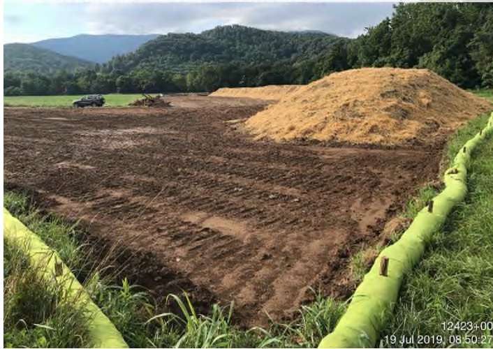
Fig. 3: ATWS 726 – Controls in place and functioning properly. Stockpiles and diversions stabilized with seed and straw.
