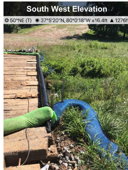
Fig. 6 Designated stream S-IJ10 ECD's and bridge in place and functioning
