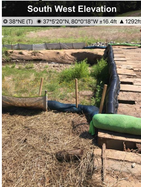
Fig. 5 Designated stream S-IJ10 ECD's and bridge in place and functioning.
