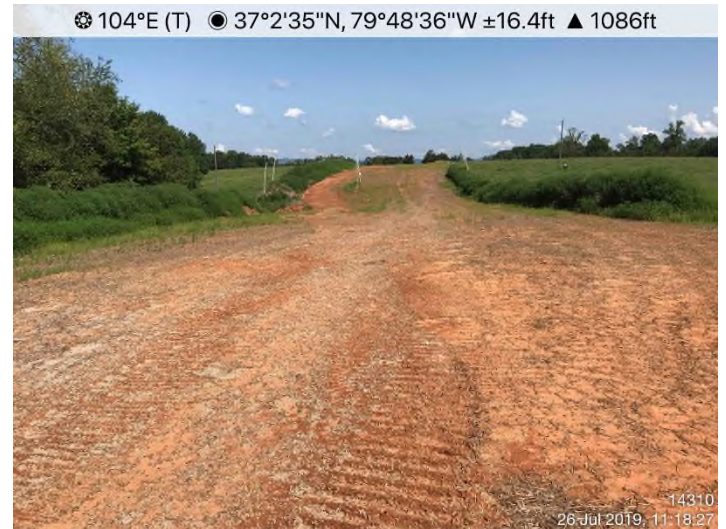
Fig. 4: STA 14310+00 – ROW stabilized with Earth Guard and millet.
