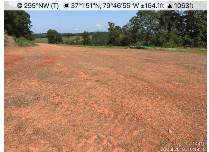
Fig. 4: STA 14310+00 – ROW stabilized with Earth Guard and millet.
