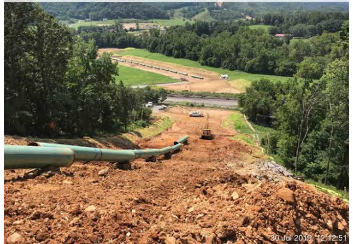
Fig. 4: STA 12415+00 – Perimeter controls in place and functioning. Topsoil piles stabilized with straw and millet.
