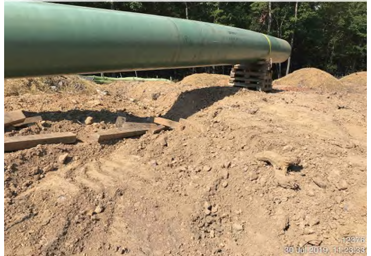
Fig. 4: STA 12415+00 – Perimeter controls in place and functioning. Topsoil piles stabilized with straw and millet.
