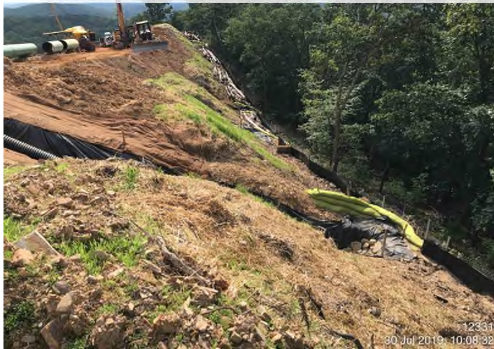
Fig. 3: STA 12331+00 – Perimeter controls and slope drains in place and functioning. Topsoil piles stabilized with straw and millet.
