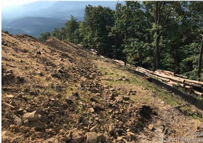
Fig. 3: STA 12331+00 – Perimeter controls and slope drains in place and functioning. Topsoil piles stabilized with straw and millet.
