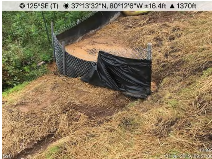
Fig. 7: STA 12483+00 – Sump maintenance needed.
