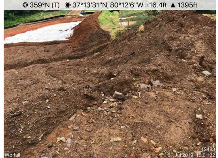
Fig. 8: STA 12483+00 – Waterbar repair needed.
