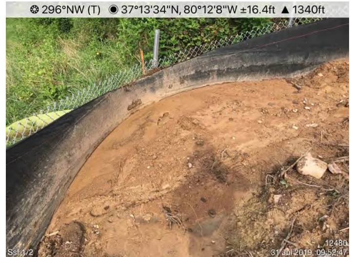
Fig. 4: STA 12481+00 – Replace damaged bridge wattle.
