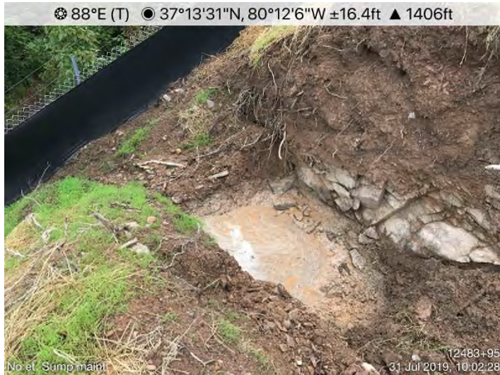
Fig. 9: STA 12483+95 – No end-treatment. Sump maintenance needed.
