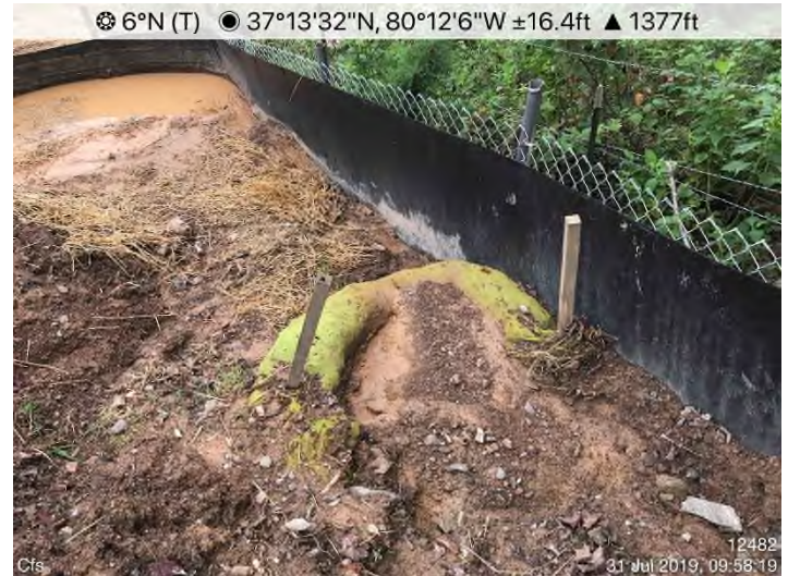
Fig. 8: STA 12483+00 – Waterbar repair needed.
