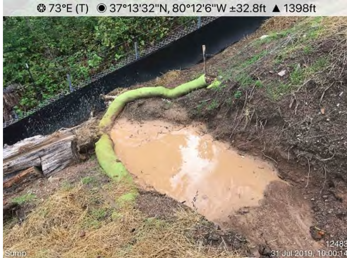
Fig. 7: STA 12483+00 – Sump maintenance needed.
