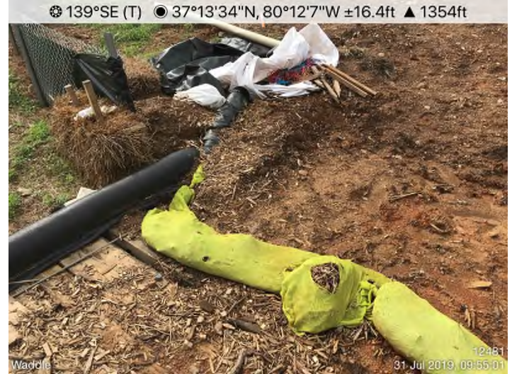
Fig. 4: STA 12481+00 – Replace damaged bridge wattle.
