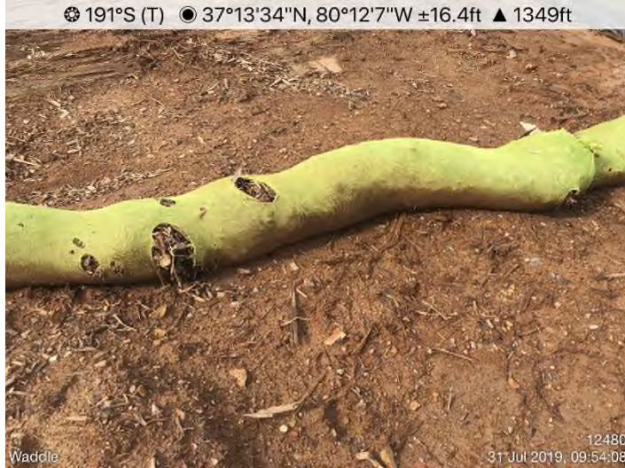
Fig. 3: STA 12480+00 – Replace damaged bridge wattle.
