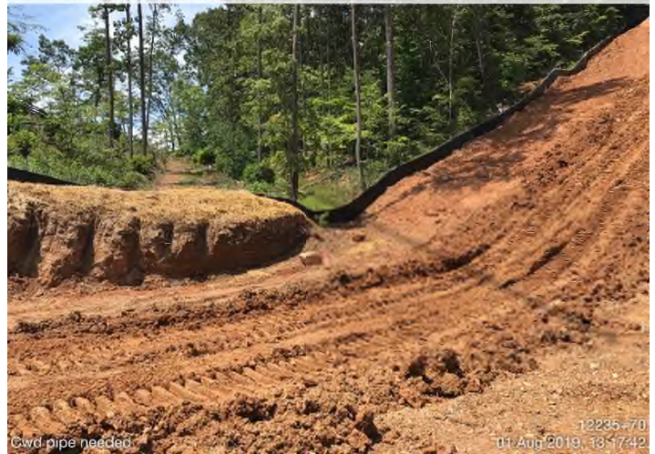
Fig. 16: STA 12532+70 – CWD needed to divert clean water around ROW.
