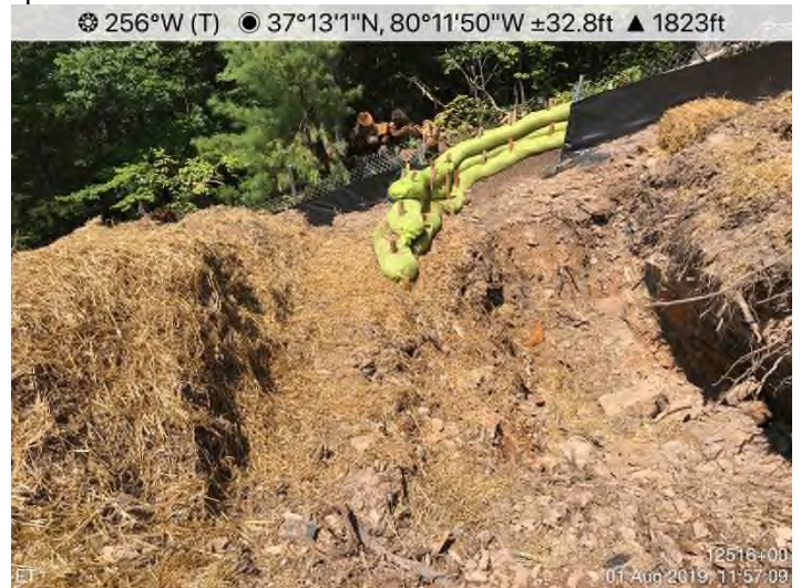
Fig. 4: Various Locations – Waterbars and End Treatments not in-compliance with the approved specifications. See MVP PSS&S MVP17 & ES42.
