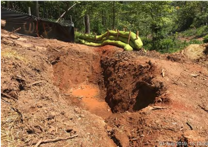
Fig. 15: Approx. STA 12533+00 to 12537+00 – Discharge directed down unprotected fill slopes. See MVP PSS&S: ES59, ES60 & ES61.
