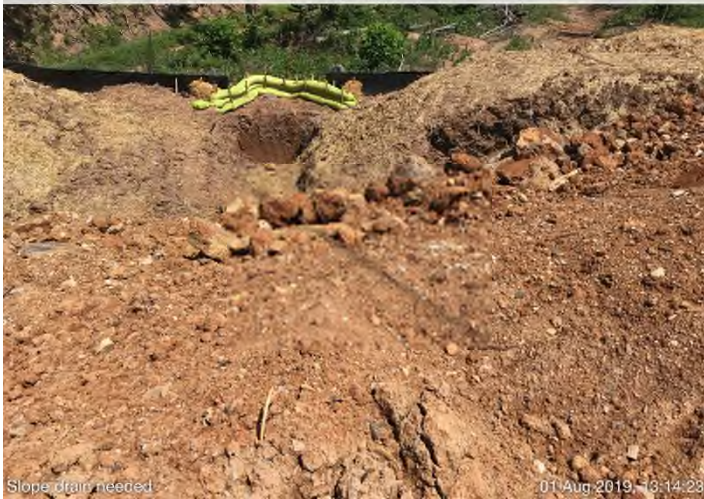
Fig. 15: Approx. STA 12533+00 to 12537+00 – Discharge directed down unprotected fill slopes. See MVP PSS&S: ES59, ES60 & ES61.
