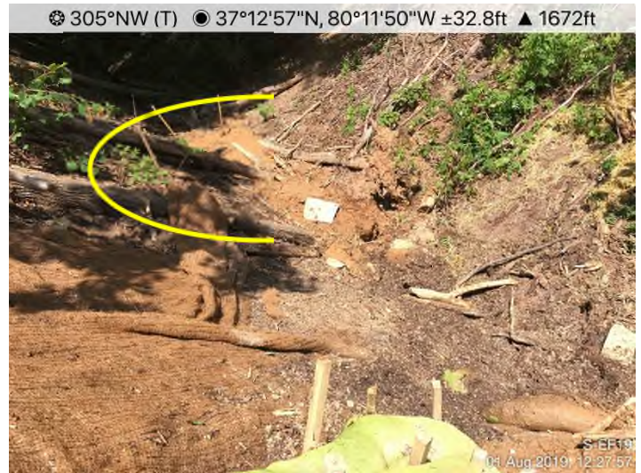
Fig. 8: Stream S-EF19 – UNT to Indian Run impacted with sediment discharge from ROW at STA 12519+41.
