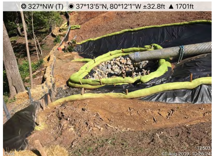
Fig. 4: Various Locations – Waterbars and End Treatments not in-compliance with the approved specifications. See MVP PSS&S MVP17 & ES42.
