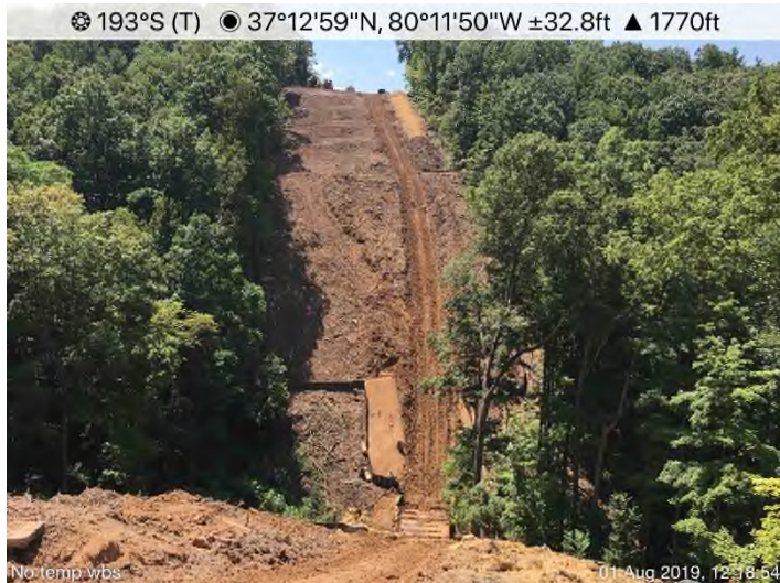
Fig. 7: Stream S-EF19 – UNT to Indian Run impacted with sediment discharge from ROW at STA 12519+41.
