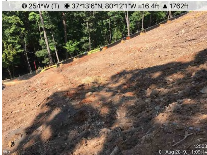
Fig. 3: Various Locations – Waterbars and End Treatments not in-compliance with the approved specifications. See MVP PSS&S MVP17 & ES42.
