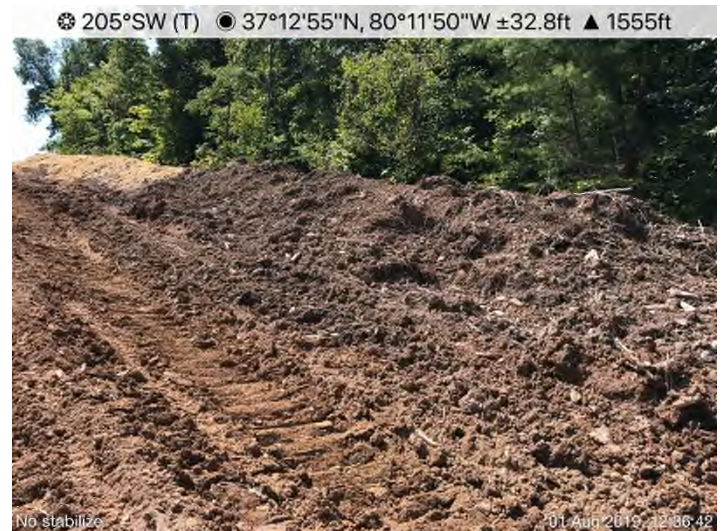
Fig. 12: Various Locations – Waterbars and End Treatments not in-compliance with the approved specifications. See MVP PSS&S MVP17 & ES42.
