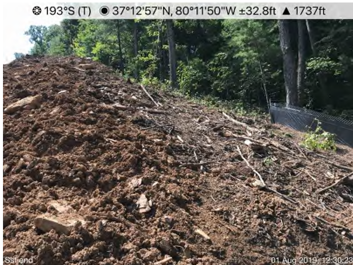
Fig. 11: Various Locations – Waterbars and End Treatments not in-compliance with the approved specifications. See MVP PSS&S MVP17 & ES42.
