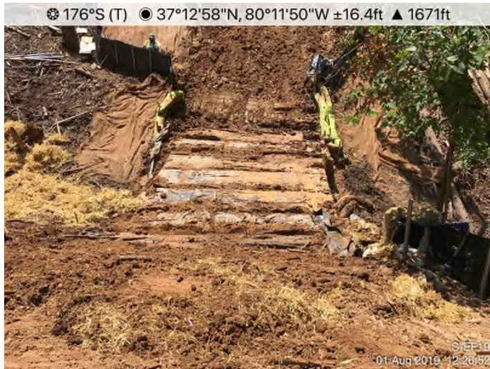
Fig. 7: Stream S-EF19 – UNT to Indian Run impacted with sediment discharge from ROW at STA 12519+41.
