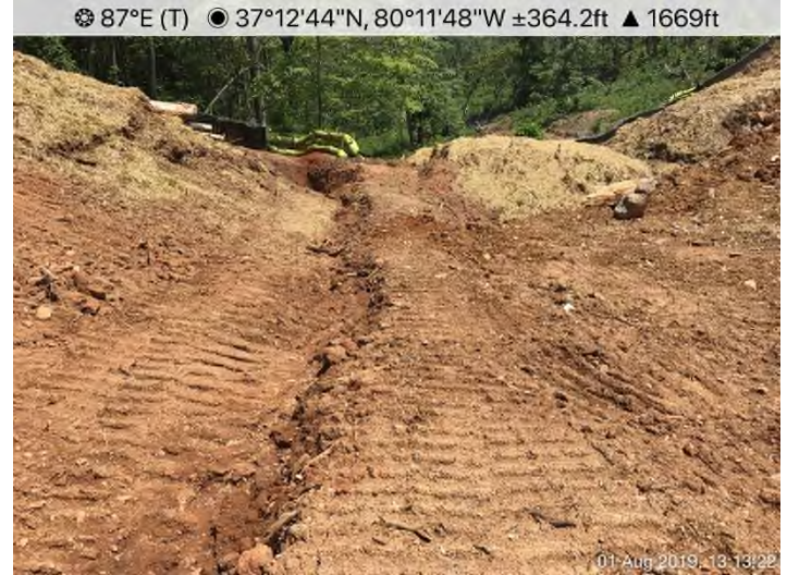
Fig. 12: Various Locations – Waterbars and End Treatments not in-compliance with the approved specifications. See MVP PSS&S MVP17 & ES42.
