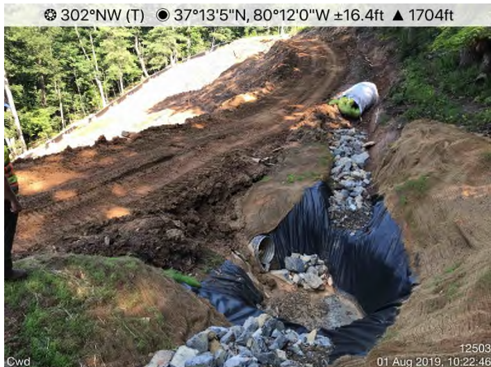
Fig. 3: Various Locations – Waterbars and End Treatments not in-compliance with the approved specifications. See MVP PSS&S MVP17 & ES42.
