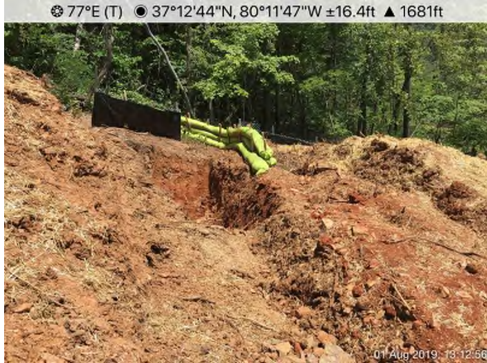
Fig. 11: Various Locations – Waterbars and End Treatments not in-compliance with the approved specifications. See MVP PSS&S MVP17 & ES42.
