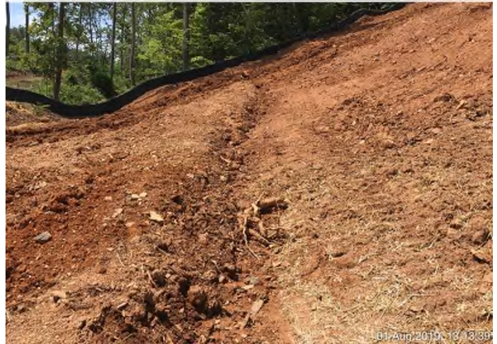
Fig. 16: STA 12532+70 – CWD needed to divert clean water around ROW.
