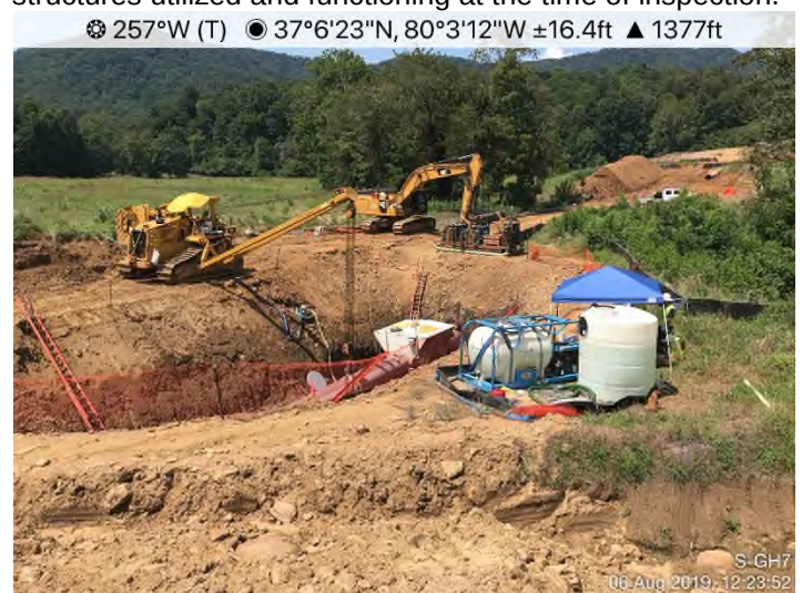
Fig. 4: Stream S-GH7 – Conventional bore ongoing. Secondary containment and controls in place. Dewatering structures utilized and functioning at the time of inspection.
