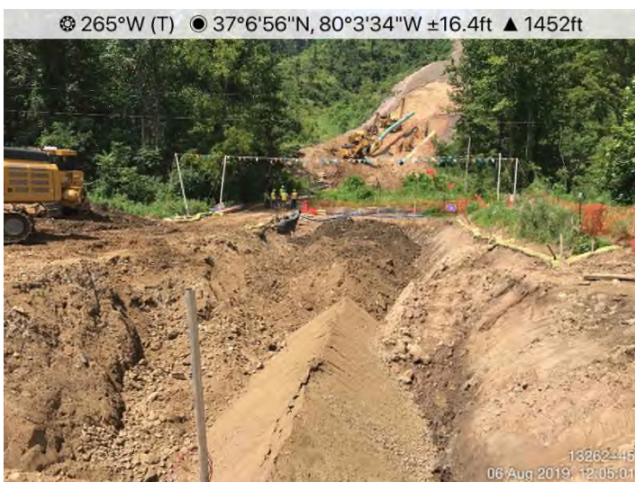
Fig. 3: Stream S-II4 – Conventional bore completed. Tie-in ongoing. Controls in place.
