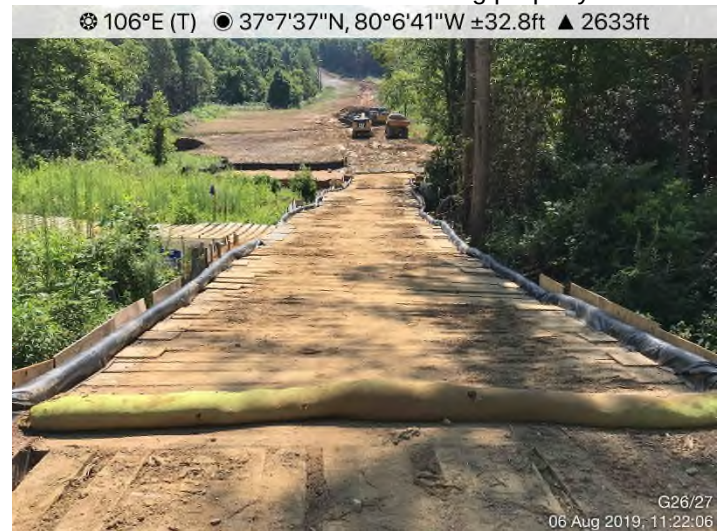
Fig. 4: Stream S-GH7 – Conventional bore ongoing. Secondary containment and controls in place. Dewatering structures utilized and functioning at the time of inspection.
