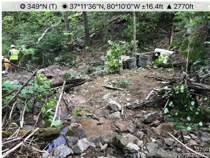
Fig. 3: Stream S-II4 – Conventional bore completed. Tie-in ongoing. Controls in place.
