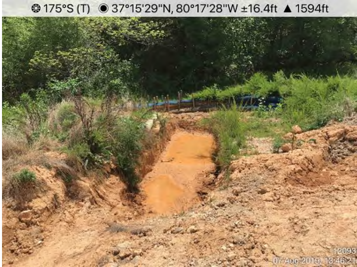
Fig. 3: STA 12093+00 – Sump maintenance needed.
