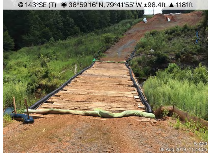
Fig. 4: Stream S-A20 – Controls in place. Sideboards and perimeter controls appear to be functioning. Area stabilized with Earth-Guard and millet.
