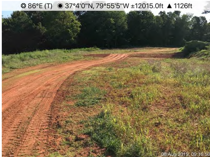
Fig. 3: STA 14695+00 – Controls in place. Area stabilized with Earth-Guard and millet.
