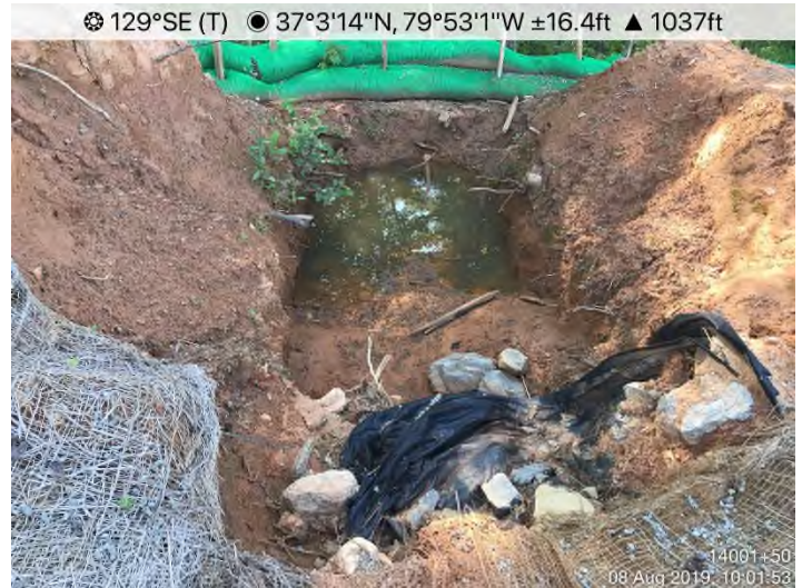
Fig. 4: Stream S-A20 – Controls in place. Sideboards and perimeter controls appear to be functioning. Area stabilized with Earth-Guard and millet.
