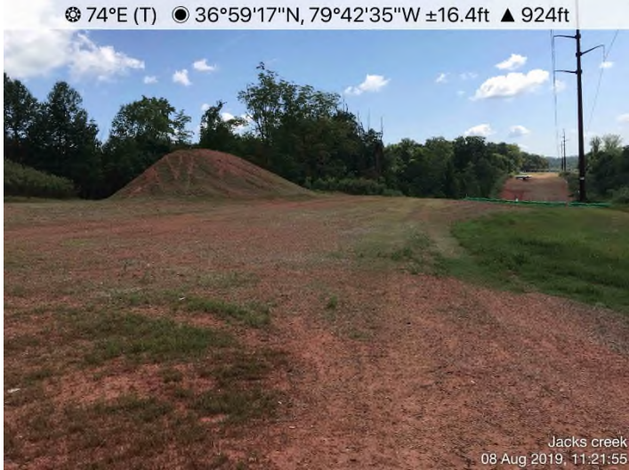
Fig. 3: STA 14695+00 – Controls in place. Area stabilized with Earth-Guard and millet.
