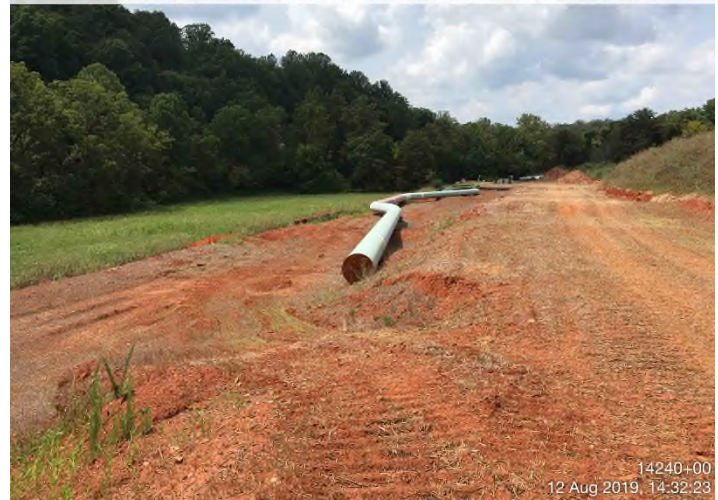
Fig. 4: STA 14240+00 – Area stabilized with Earth-Guard, millet and straw. Controls in place and functioning. No observed sediment off ROW.
