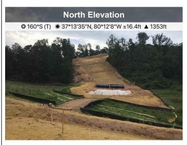
Fig. 4. Near St12482+67 stabilization has been applied.
