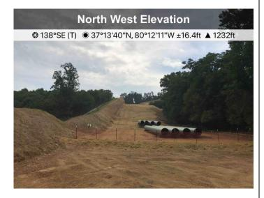
Fig. 3. Near St12181+00 ECD's are in place and stabilization has been applied.
