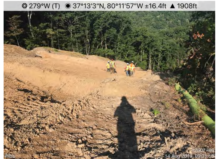
Fig. 4: Stream S-EF19 – Controls in place along stream S-EF19. SSF entrenched properly and stabilized with erosion matting.
