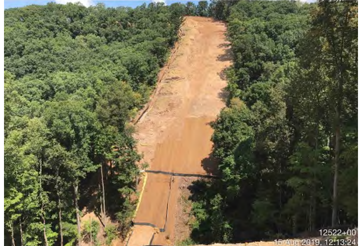
Fig. 4: STA 12504+00 – Controls in place. Sideboards for CWD crossing installed. Area stabilized with erosion matting and millet.
