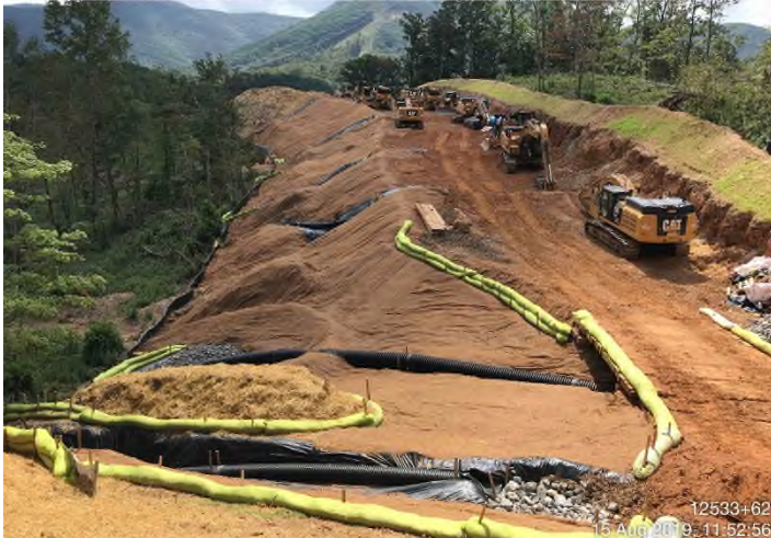
Fig. 3: STA 12515+30 – Controls in place. Berms stabilized with straw and millet. Waterbars installed full length of ROW and connected to sumps and end-treatments.
