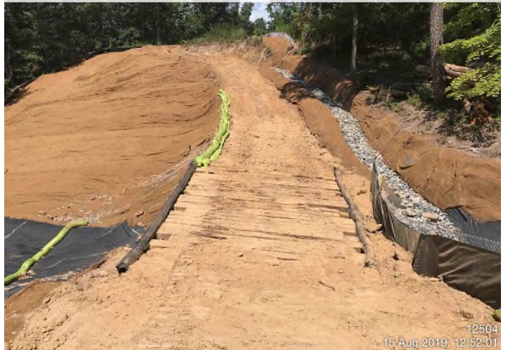
Fig. 4: STA 12504+00 – Controls in place. Sideboards for CWD crossing installed. Area stabilized with erosion matting and millet.
