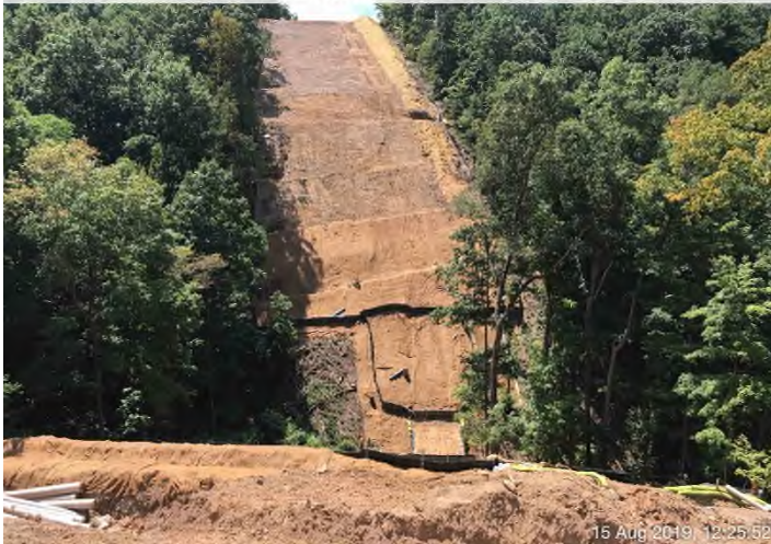
Fig. 3: STA 12515+30 – Controls in place. Berms stabilized with straw and millet. Waterbars installed full length of ROW and connected to sumps and end-treatments.
