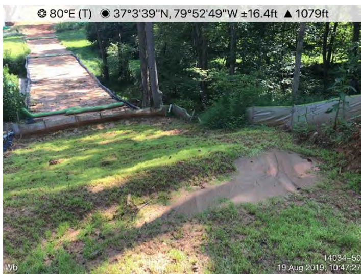
Fig. 3: STA 14033+50 to 14034+50 – Maintain waterbars.
