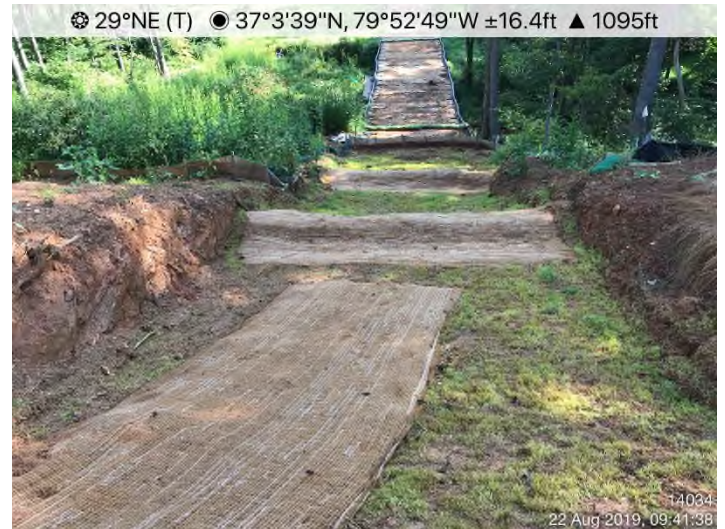
Fig. 4: STA 14034+00 – Waterbars repaired and stabilized with erosion fabric and seed.
