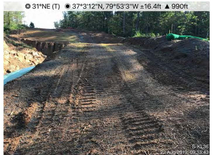
Fig. 4: STA 14034+00 – Waterbars repaired and stabilized with erosion fabric and seed.
