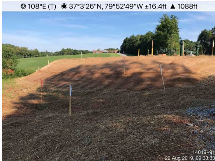
Fig. 3: STA 14019+91 – Area stabilized with erosion fabric, seed and straw.
