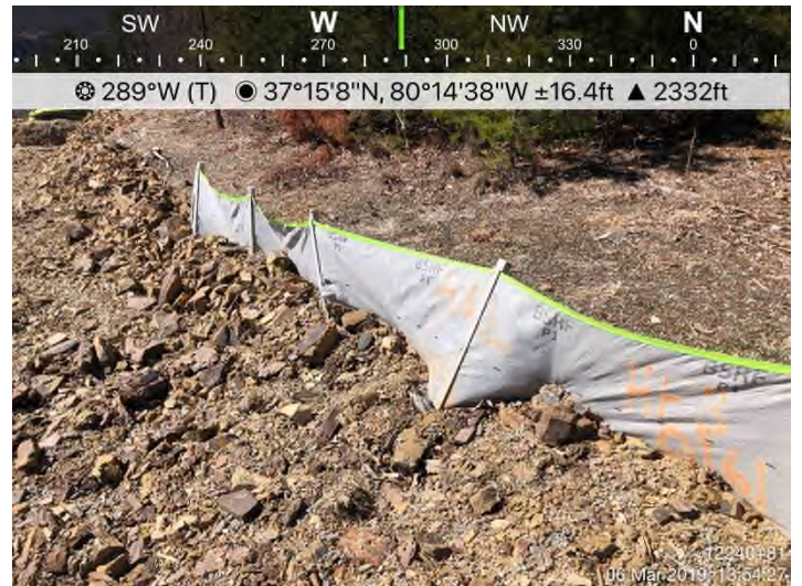
Fig. 8: STA 12240+81 – P1 needs maintenance.
